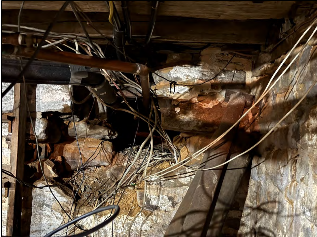
Plate 134. Access point between main building and southern wing, facing south.
