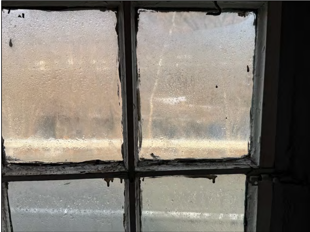
Plate 276. Room 13, Detail of window muntin, facing north.
