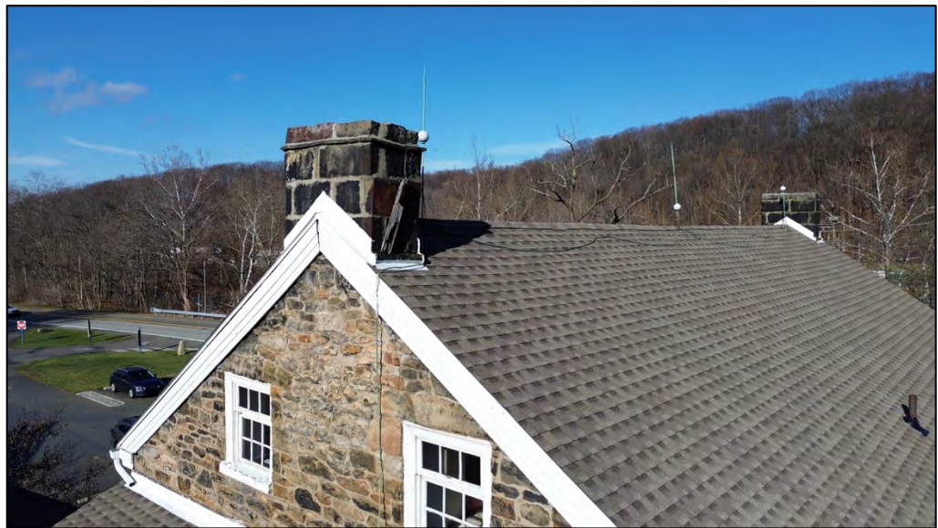
Plate 64. Chimney 3, facing northwest.
