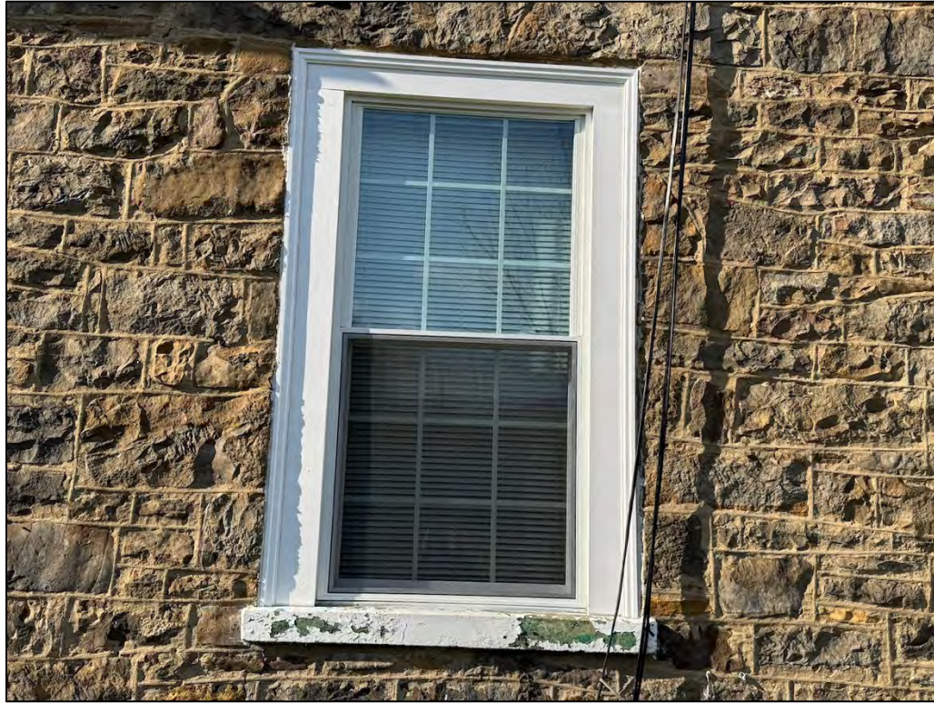
Plate 22. Detail of typical beaded mortar joint, east elevation.
