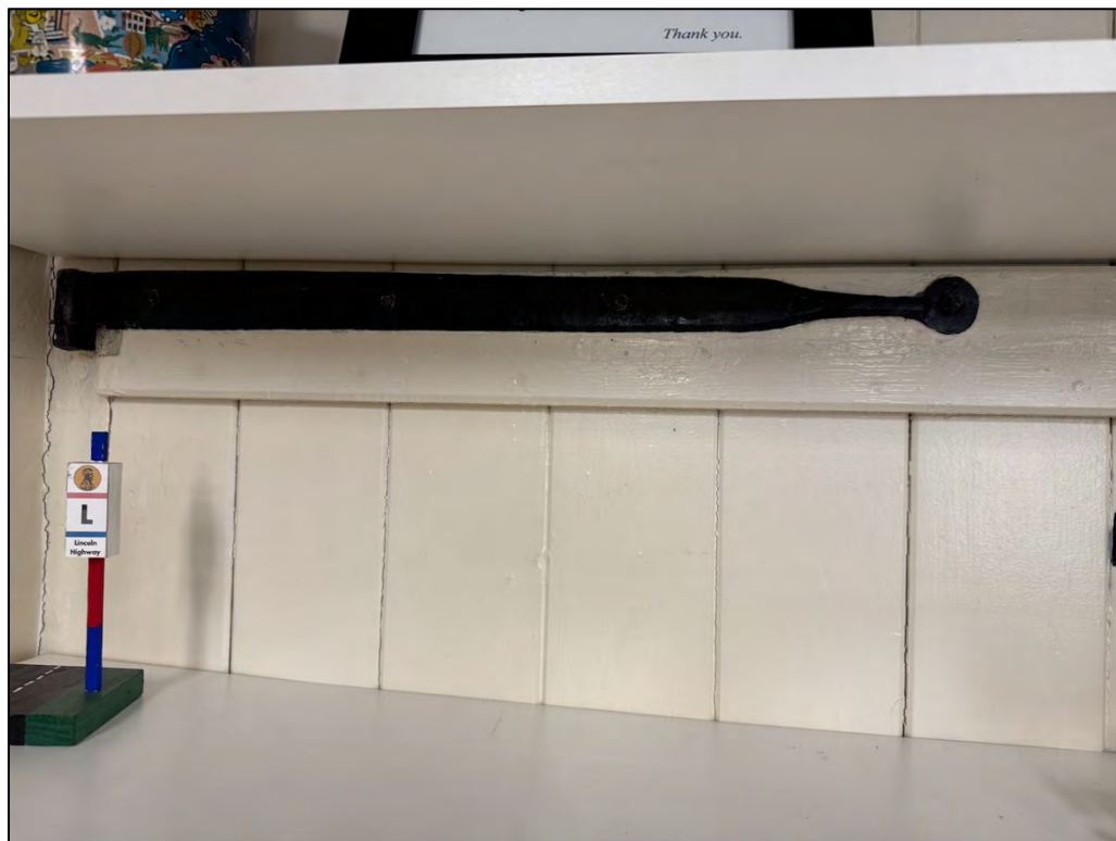
Plate 241. Detail of original hardware in Tot Room, facing south.
