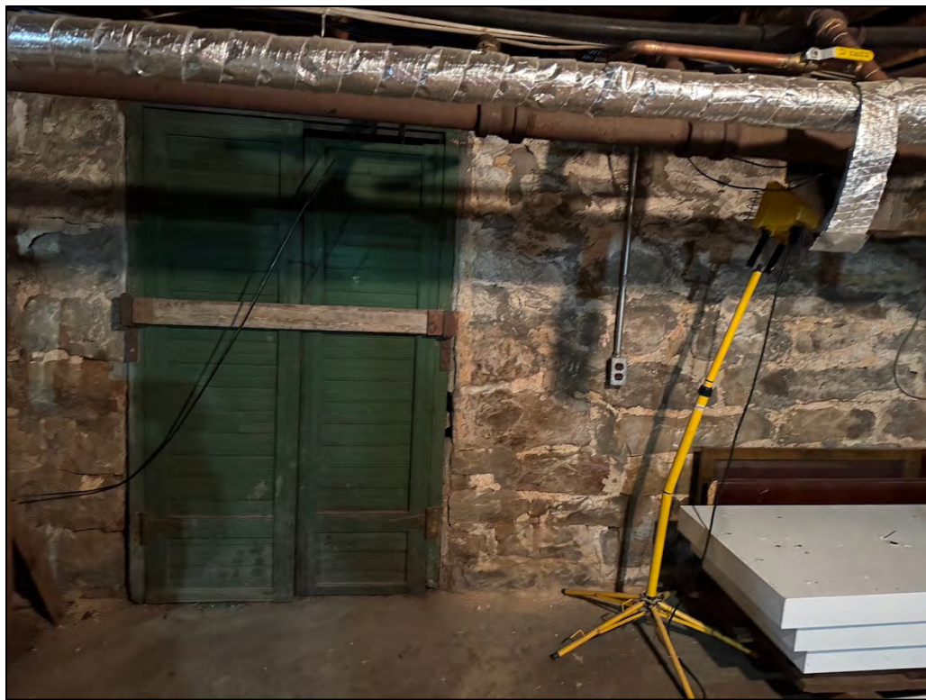
Plate 128. Exterior door which is currently inaccessible. The door may provide access to the bulkhead.
