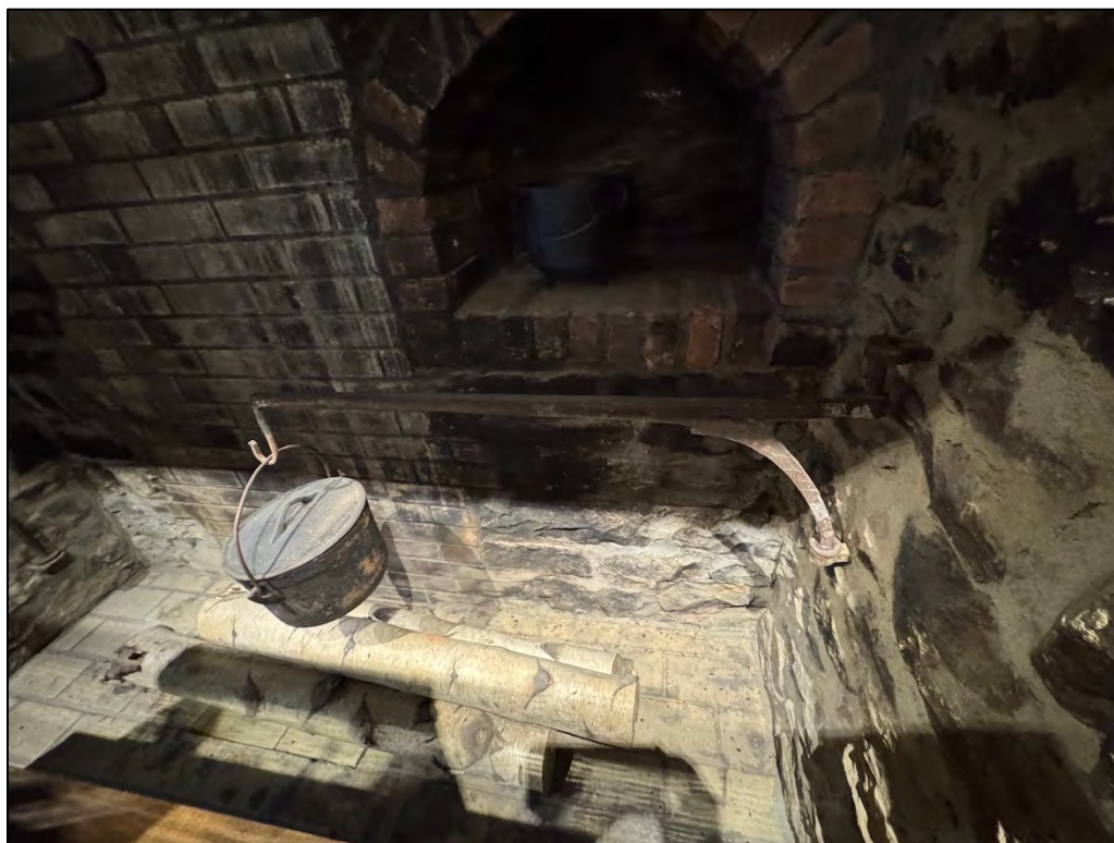
Plate 225. Interior of fireplace with bake oven, facing south.
