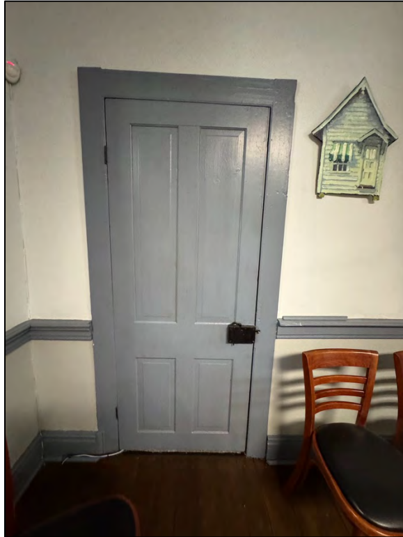
Plate 170. Parlor door, facing north.
