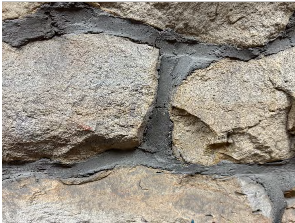
Plate 138. Typical non-historic mortar joint, facing east.
