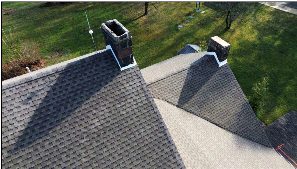
Plate 66. Chimney 3 and Chimney 4, facing southeast.
