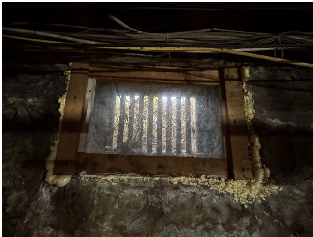
Plate 131. Typical basement window, facing east.
