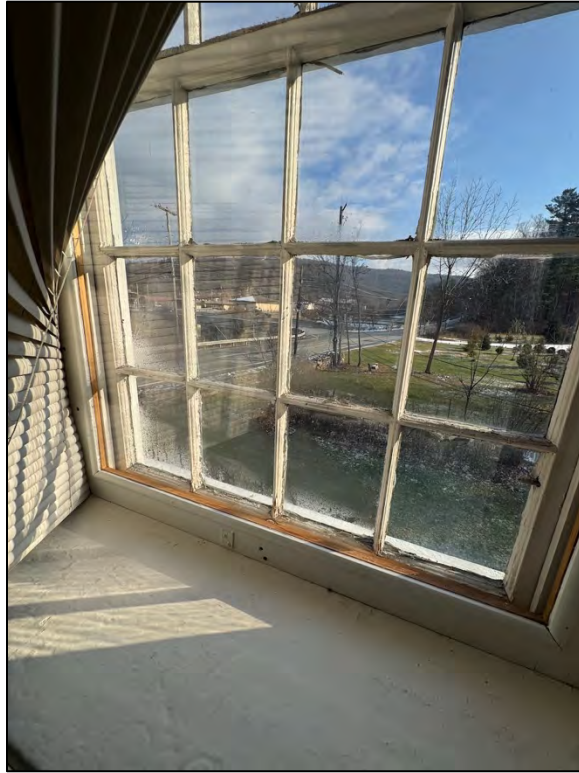
Plate 295. Lower sash of window 2-11, facing east. Note interior storm window.
