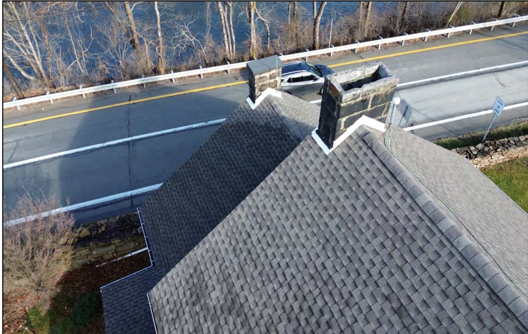
Plate 59. Chimneys 1 (covered) and 2 (uncovered), facing north.
