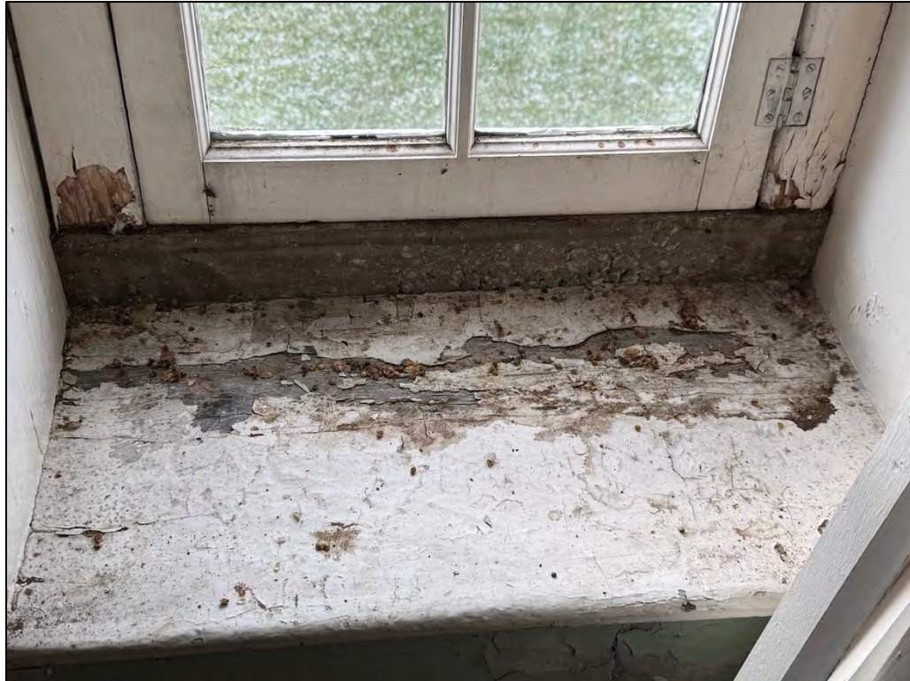
Plate 324. Room 18, south wing upper storage area, southeast window.
