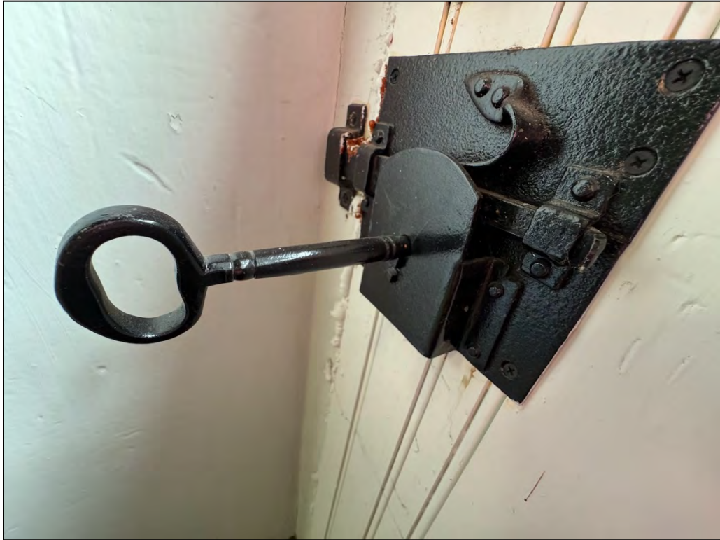
Plate 91. Assumed original box lock and key (installed on a replacement door).
