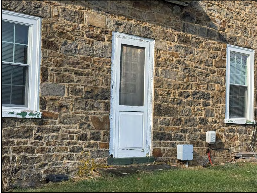
Plate 102. Southernmost door on east elevation.
