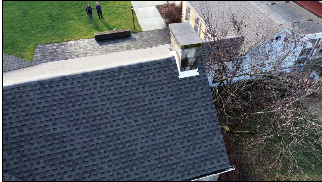
Plate 73. Chimney 5, facing south.
