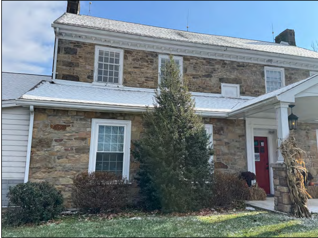
Plate 42. West elevation, facing east. Typical gutter and downspout configuration.
