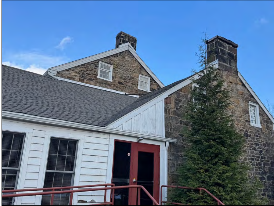
Plate 112. View of the south elevation door.
