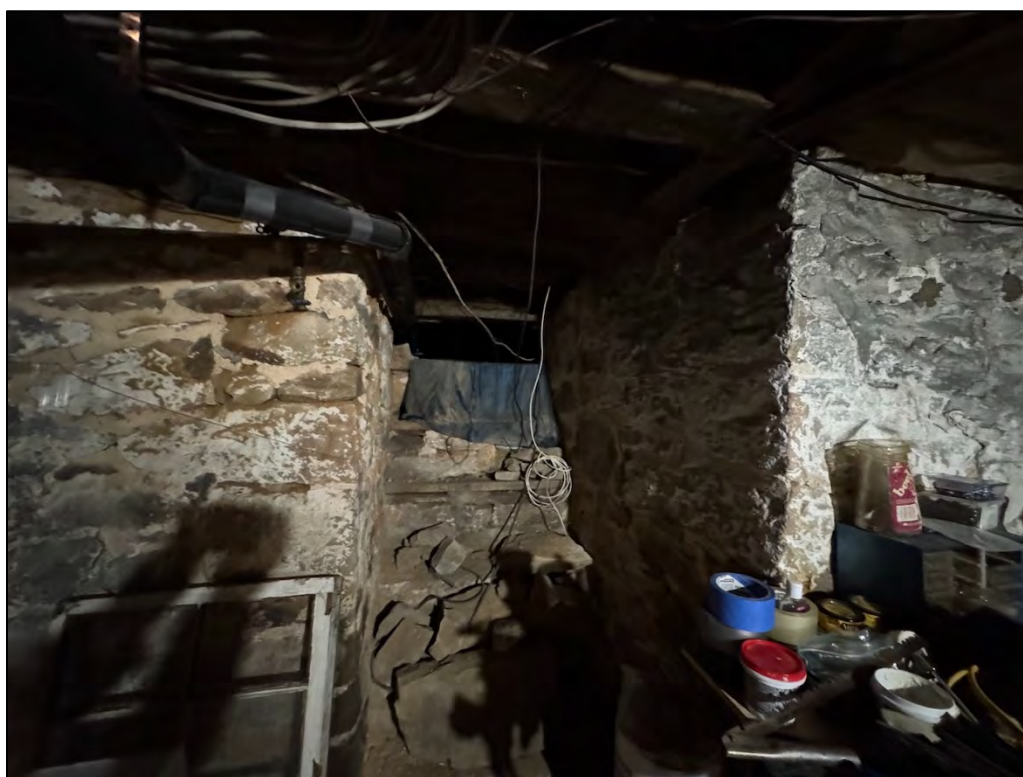
Plate 132. Access to the crawl space in the southern wing, facing south.
