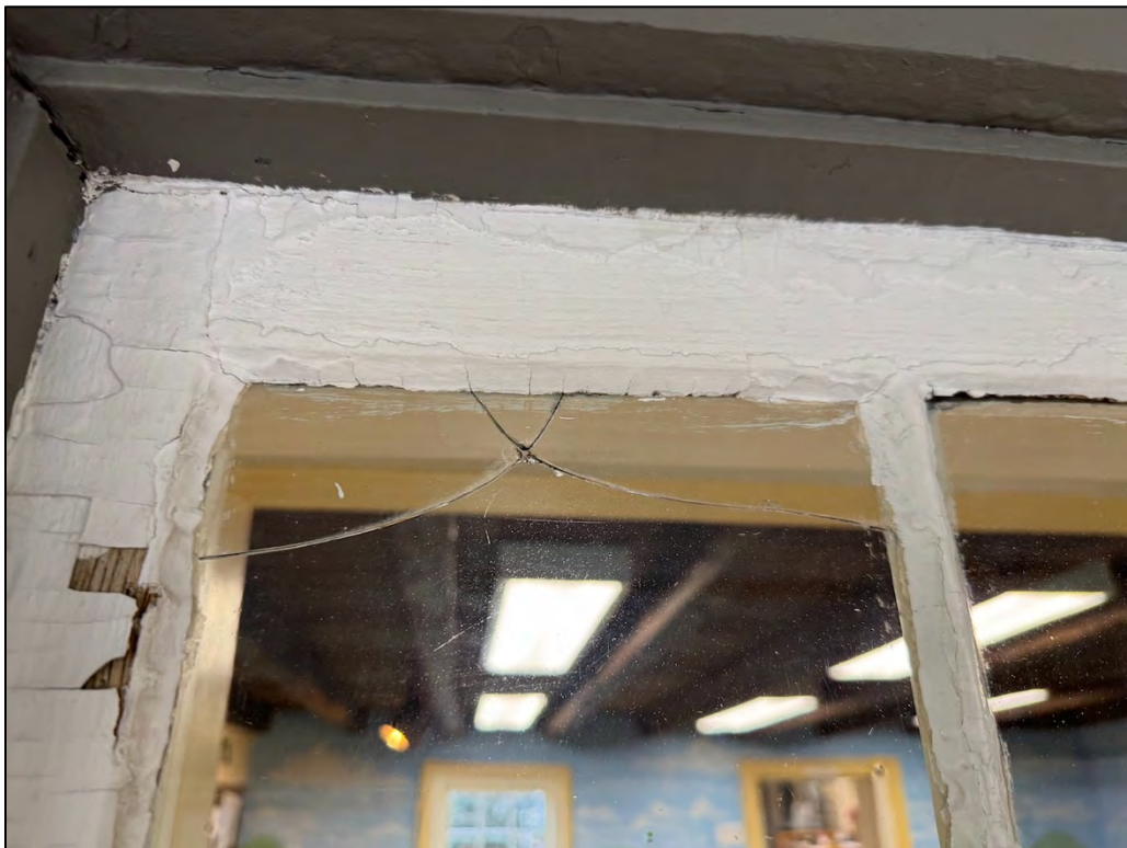
Plate 258. Typical condition of historic window, facing north.
