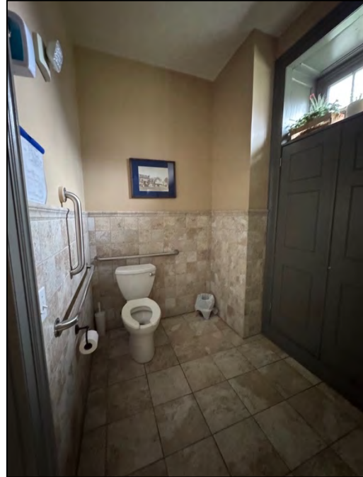
Plate 193. Interior of bathroom, facing northeast.
