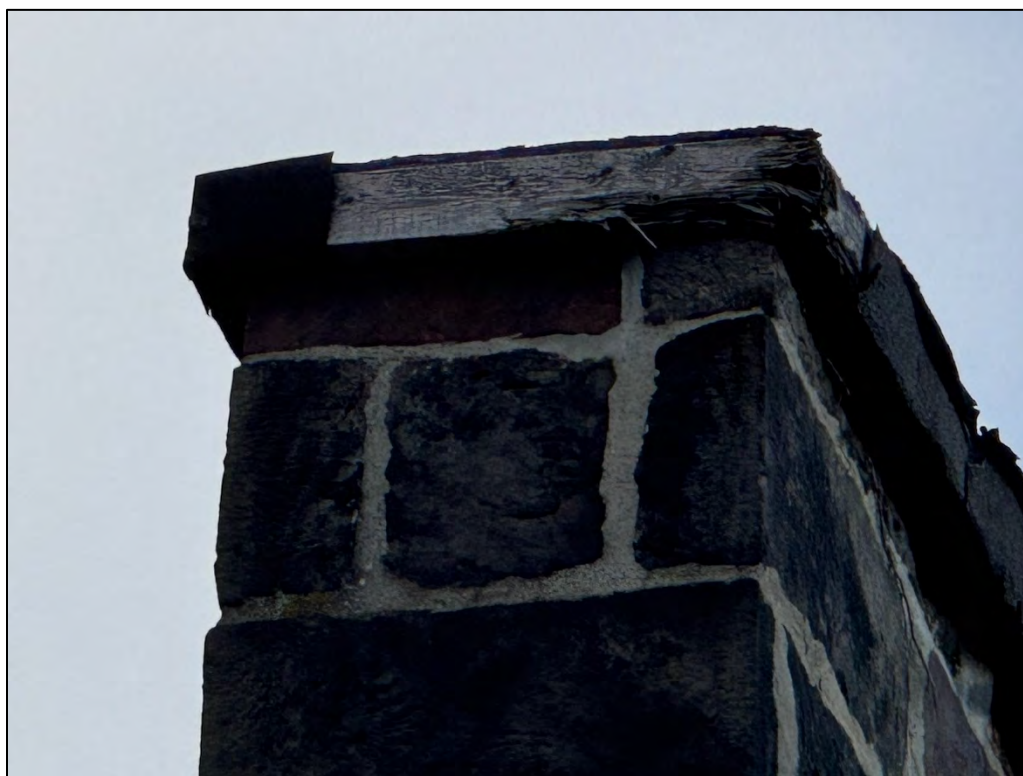
Plate 68. Detail of Chimney 4. Note the cap is constructed of wood wrapped in tar paper. Facing northeast.
