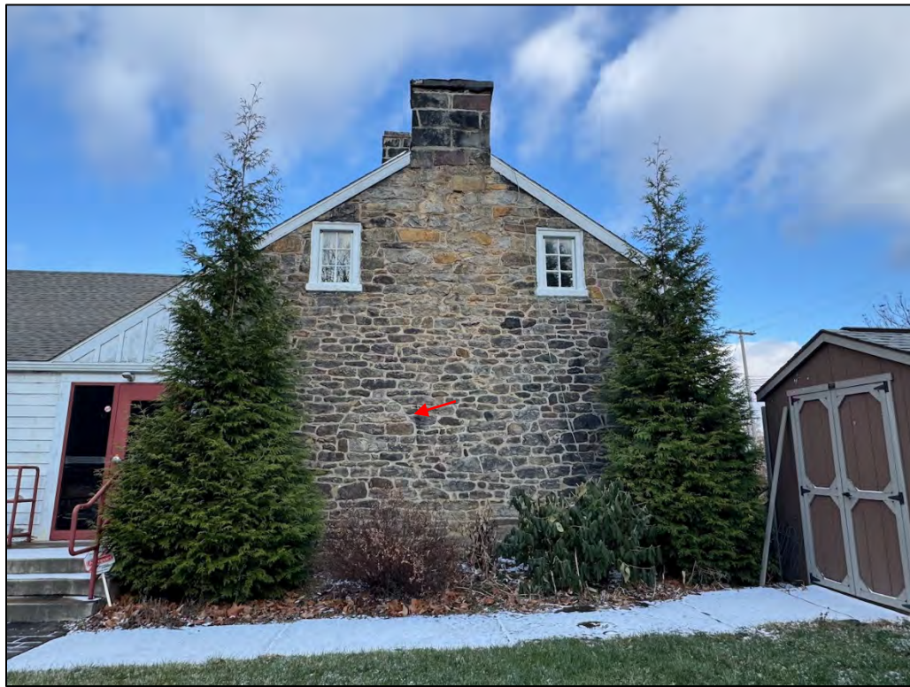
Plate 30. South elevation. Note the ghost mark of the oven which was previously removed.
