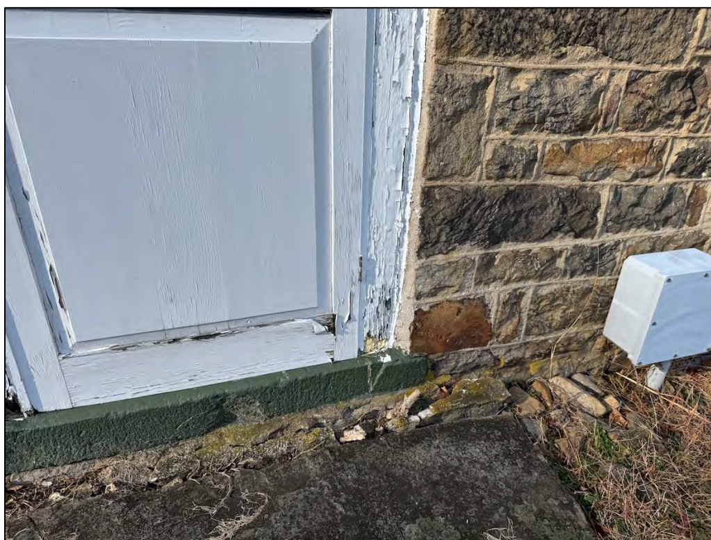
Plate 106. Lower right (north) corner of door. Note flaked paint.
