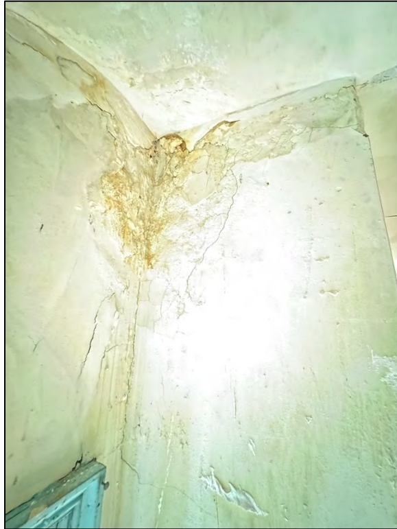
Plate 350. Plaster walls facing southwest.
