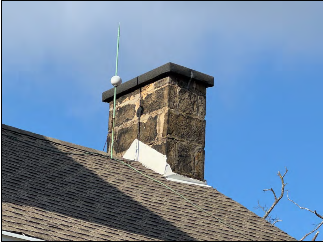
Plate 57. Chimney 1, facing northwest.
