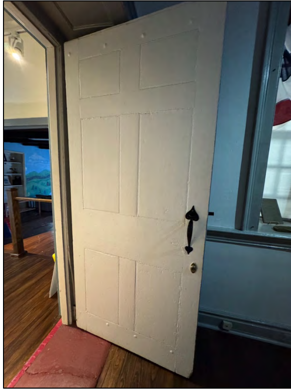
Plate 197. Door from Convoy Room to hallway, facing west. Note the rivets at the top and bottom of the door.
