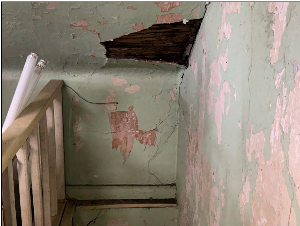
Plate 328. Room 18, south wing upper storage area, facing west.
