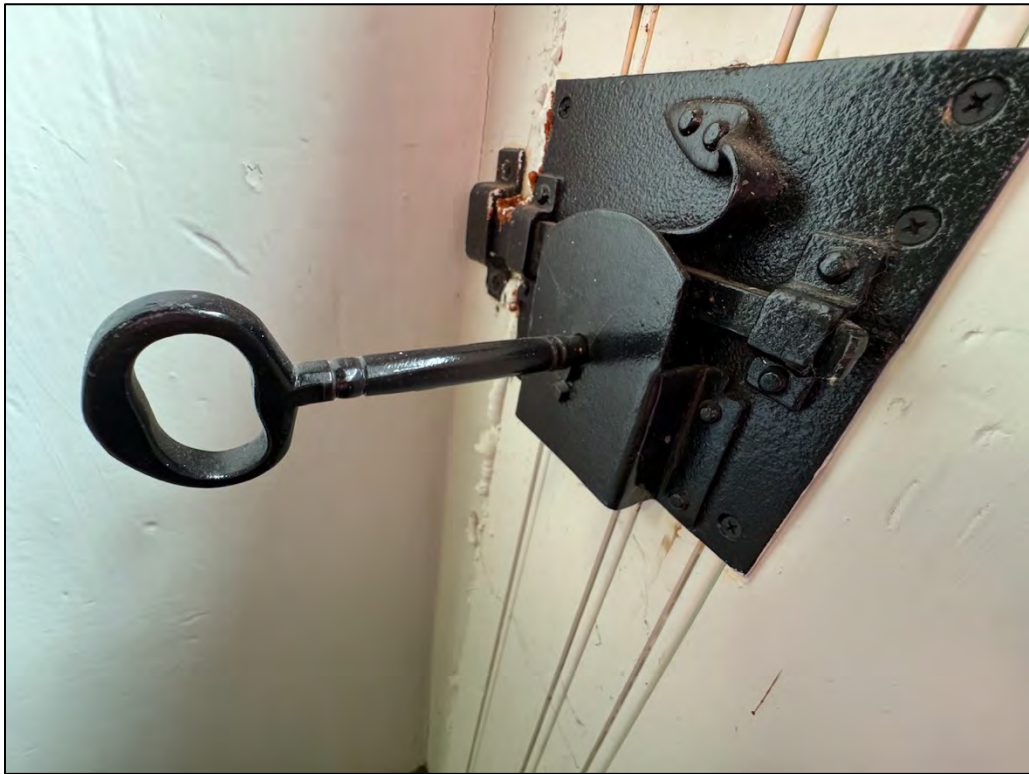
Plate 158. Entry hardware on door, note the rivets.
