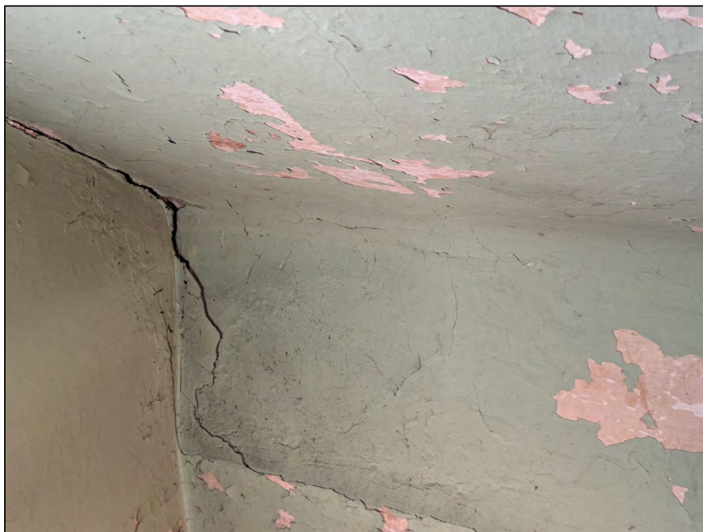
Plate 325. Room 18, south wing upper storage area, facing west.
