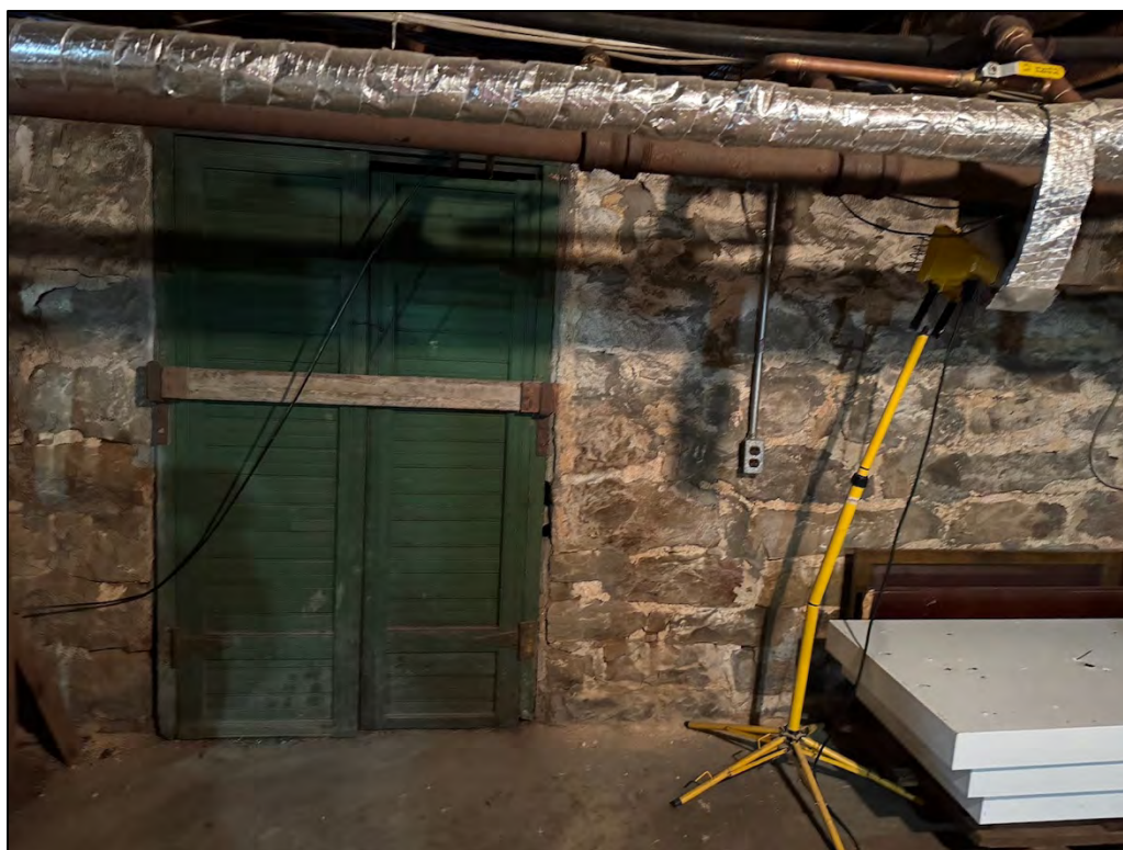
Plate 38. Basement foundation, facing south
