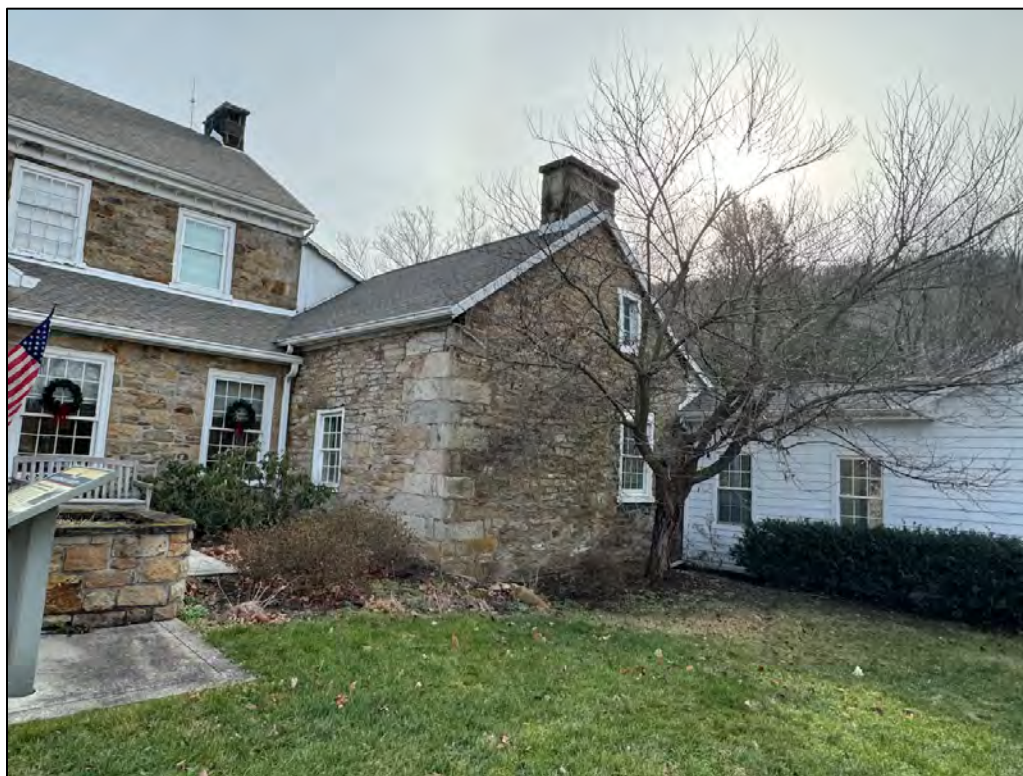
Plate 32. Tavern ell addition, facing southeast. The ghost mark of the beehive oven has been hidden through repointing.
