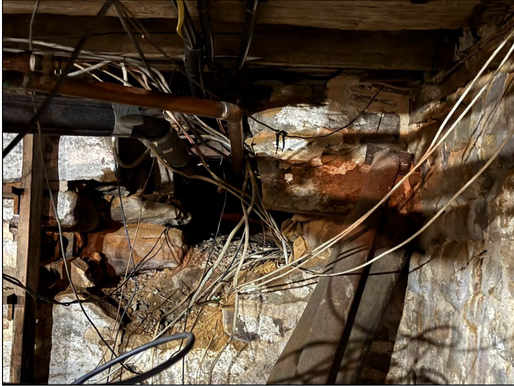
Plate 39. Hole cut through south wall in foundation, facing south.
