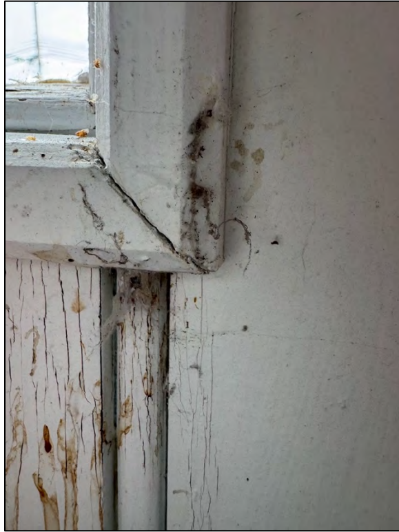
Plate 93. Detail of southern corner of window in door, facing northeast. Note staining from insect activity.
