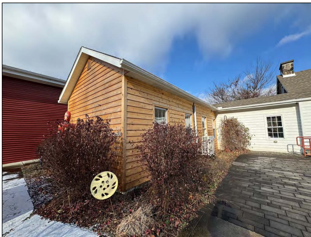
Plate 49. Newly re-sided gallery with new gutters and downspouts.
