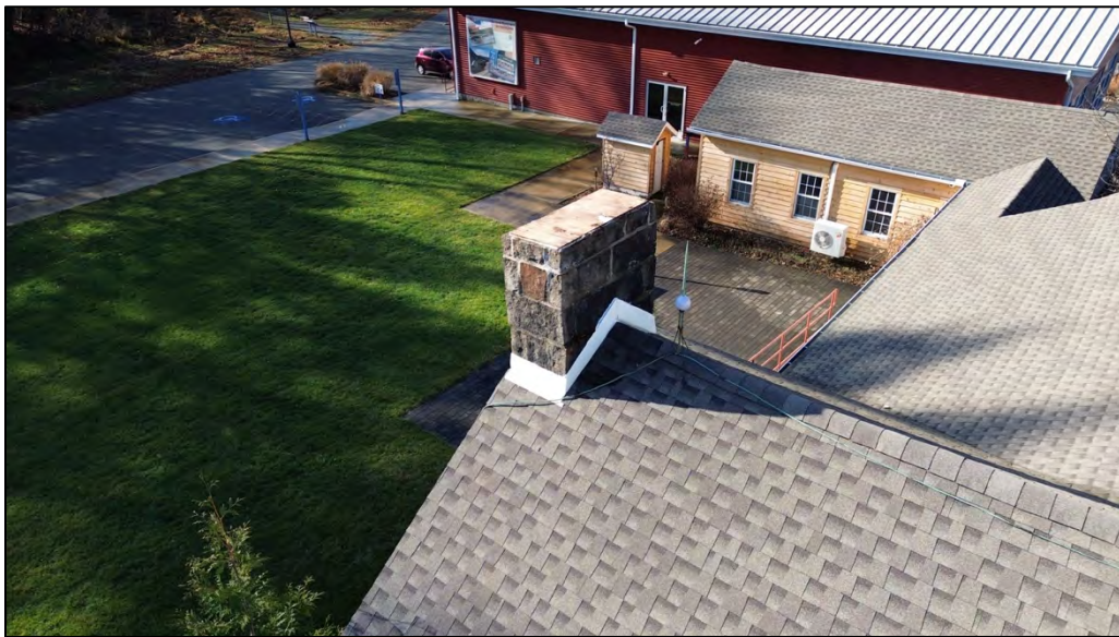
Plate 70. Aerial photo taken December 10, 2025 showing plywood cover.
