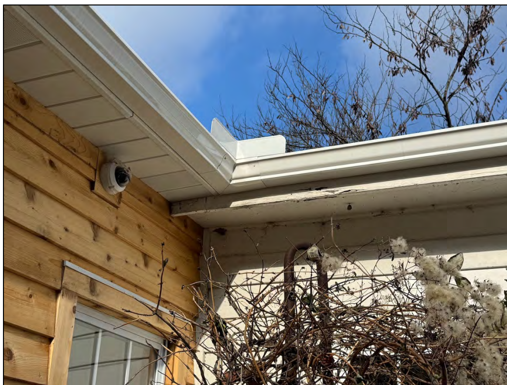
Plate 50. New gutter intersection.
