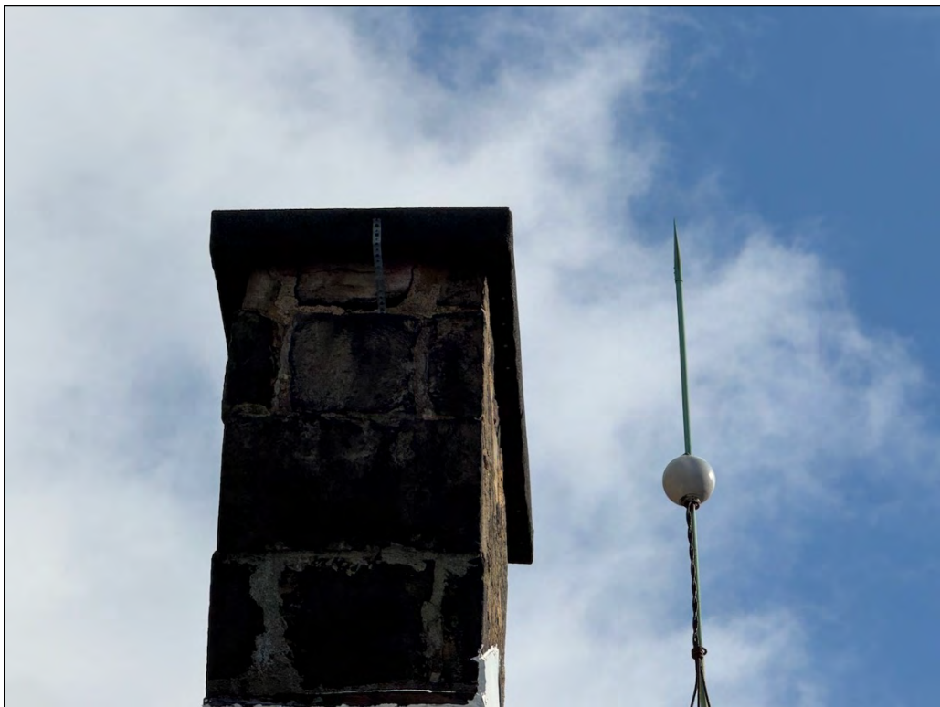
Plate 58. Chimney 1, facing northeast.
