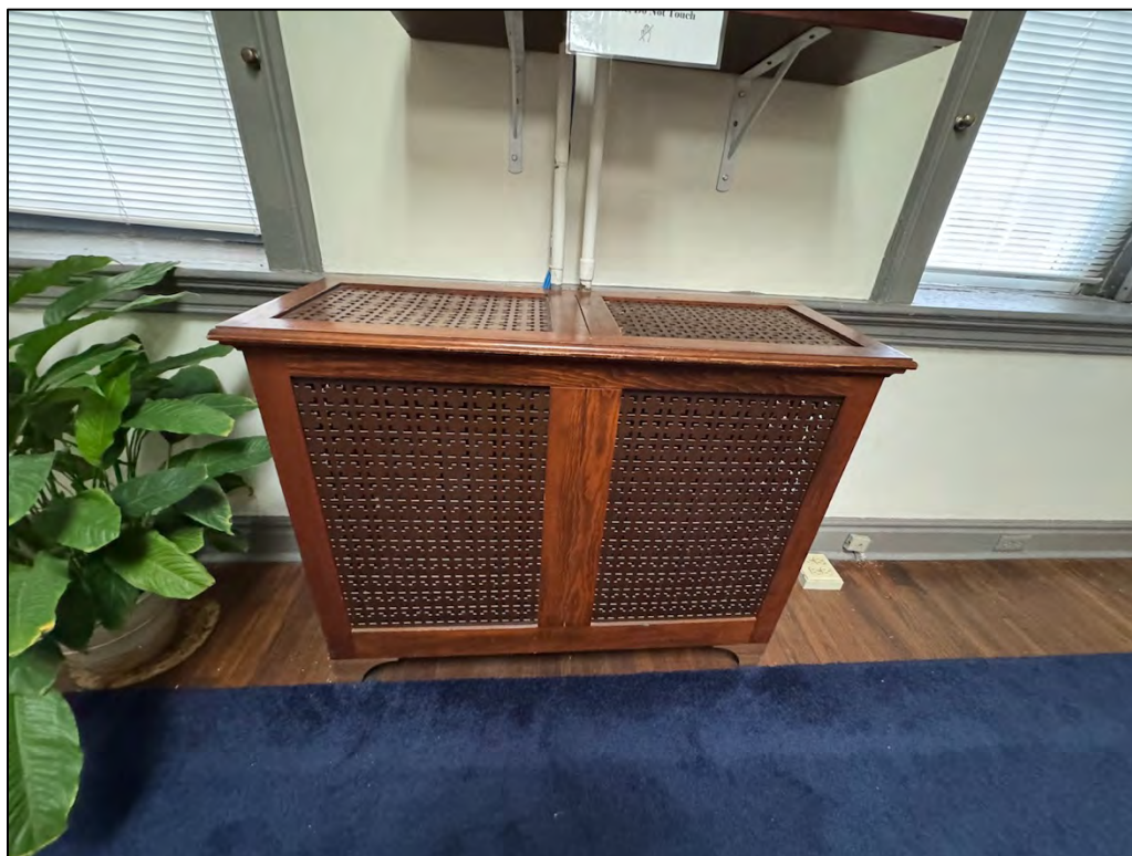
Plate 212. Freestanding radiator and cover, facing east.
