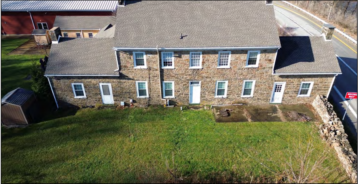
Plate 40. East elevation, facing west.
