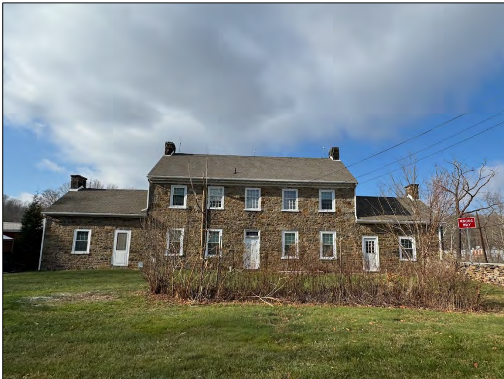
Plate 21. East elevation, facing west.
