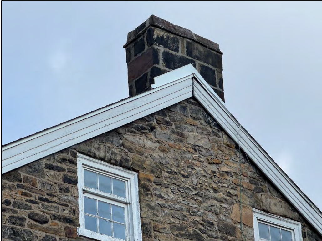
Plate 62. Chimney 3, facing northeast.
