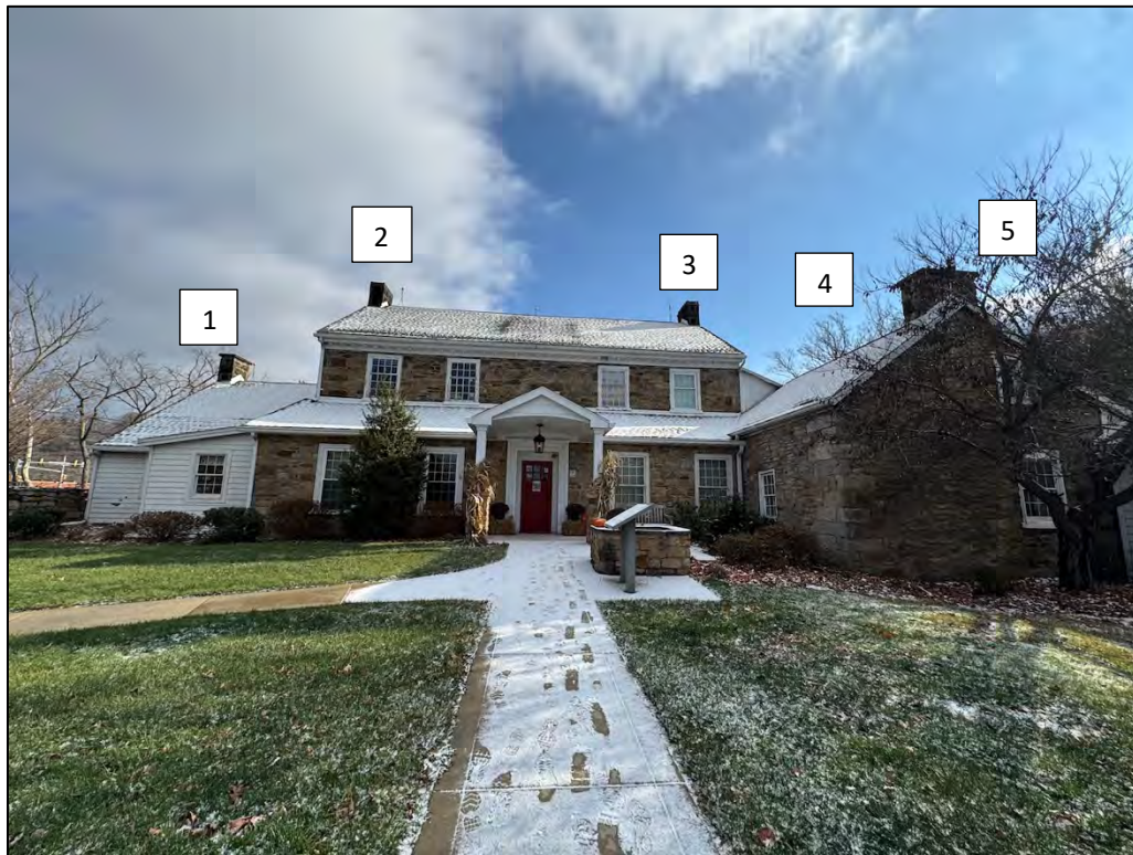
Plate 56. West elevation, facing east. Note there are five existing chimneys (chimney #4 not visible).
