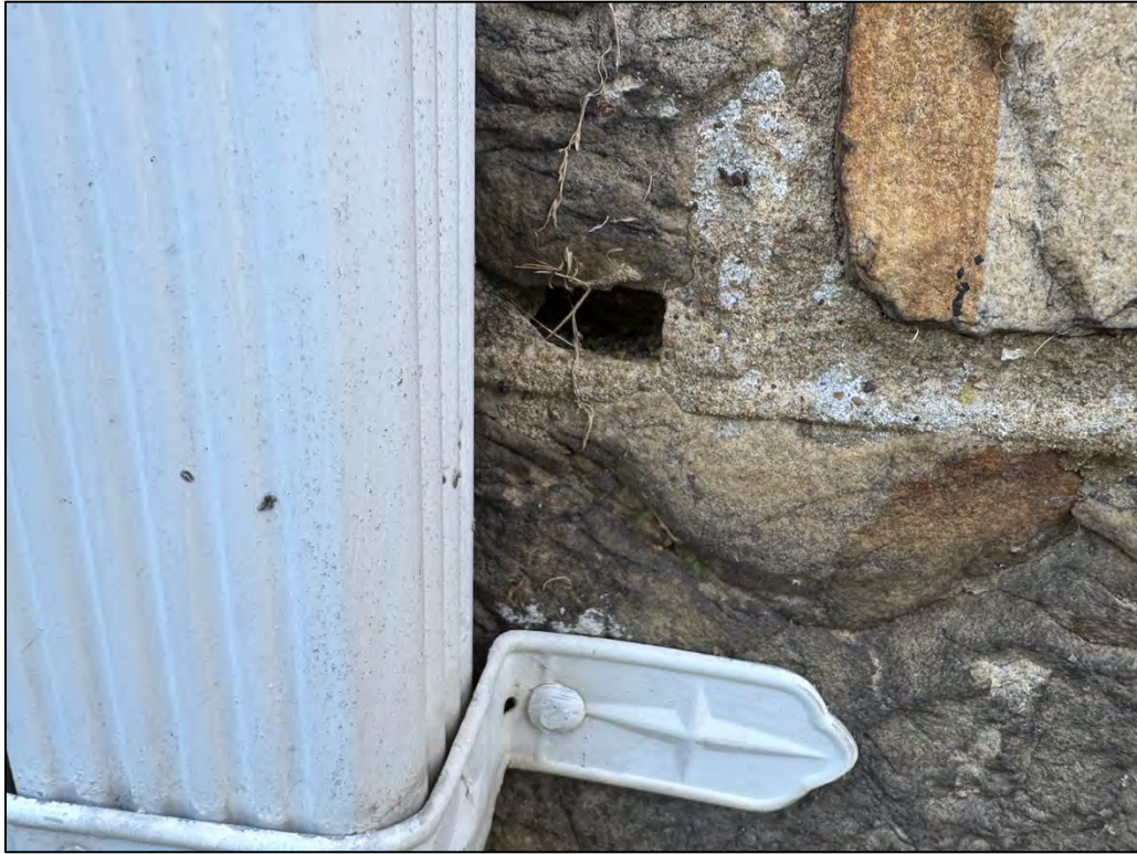
Plate 28. Missing mortar
