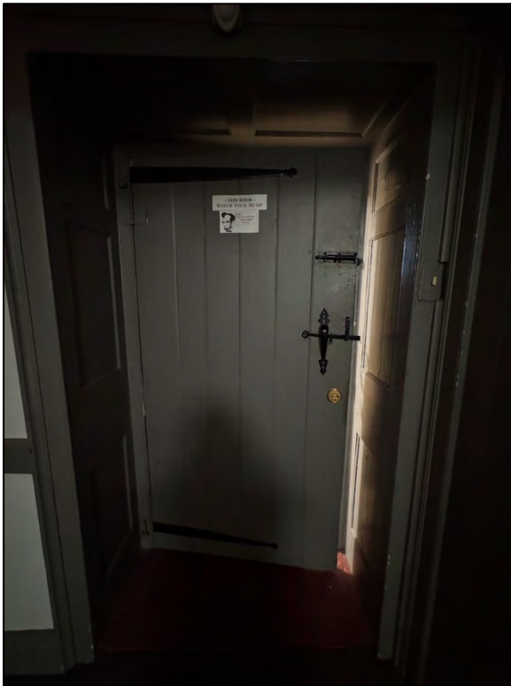
Plate 175. Rear of historic rear entry door, facing west toward the lobby. Note the hinge straps.
