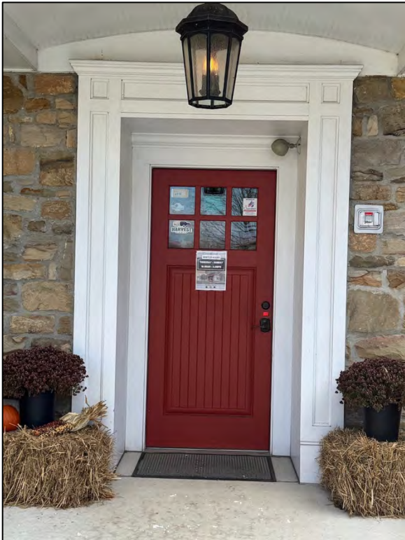
Plate 114. Front entry on west elevation.
