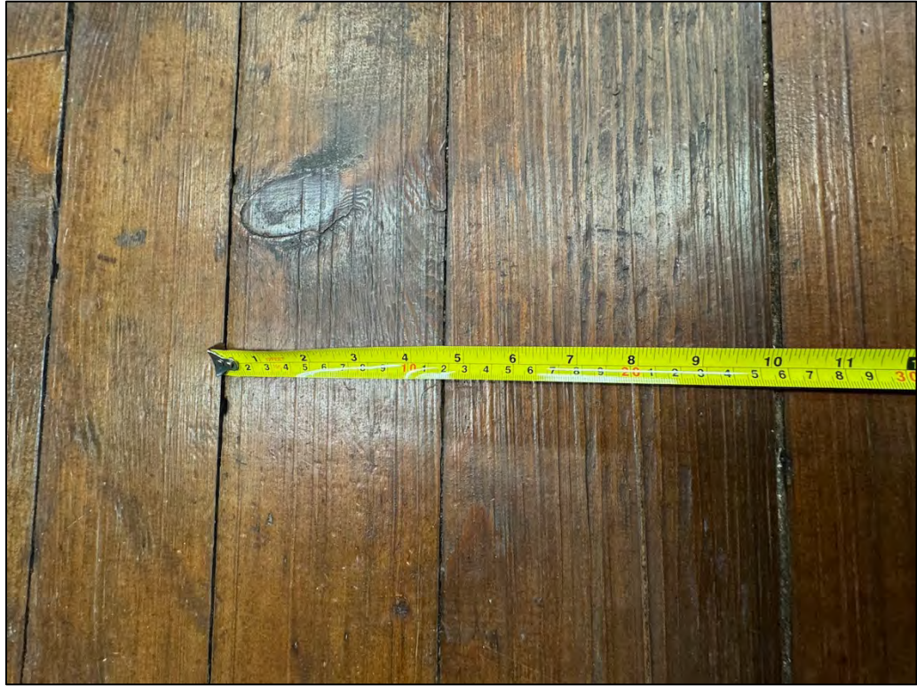
Plate 234. Typical flooring widths in Tot Room.
