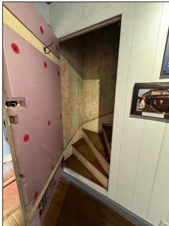
Plate 222. Ship Room hidden staircase, facing north.
