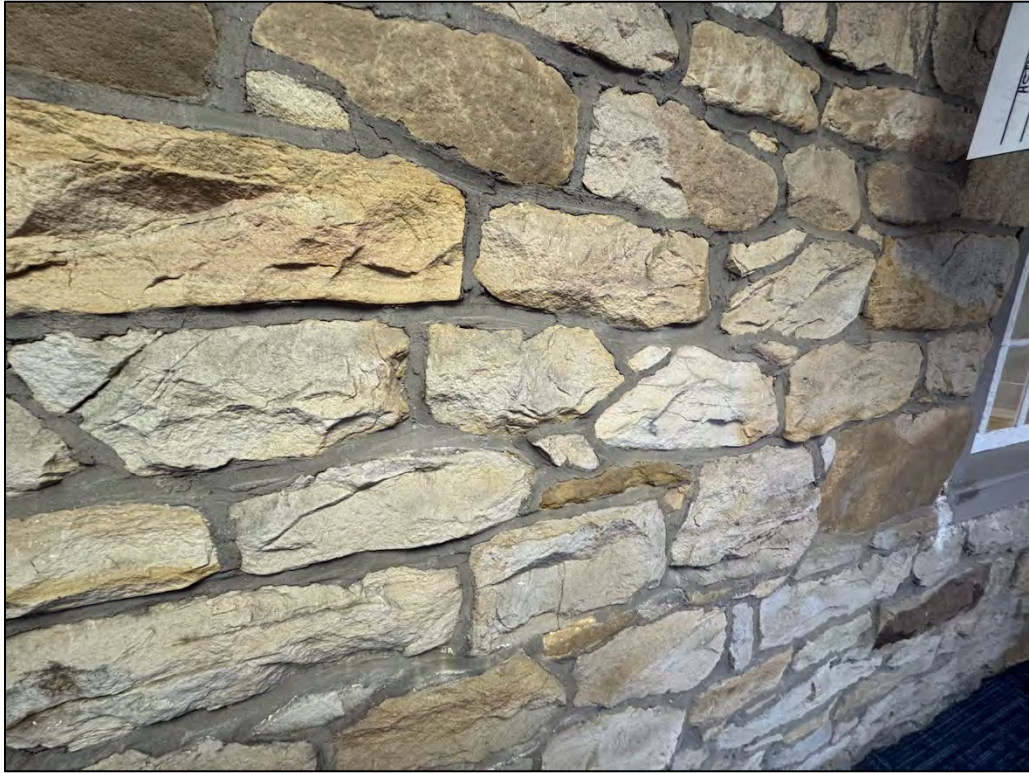
Plate 257. Typical repointing job in Postcard Corridor, facing north.
