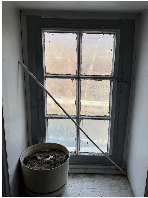
Plate 275. Room 13 window, facing north.
