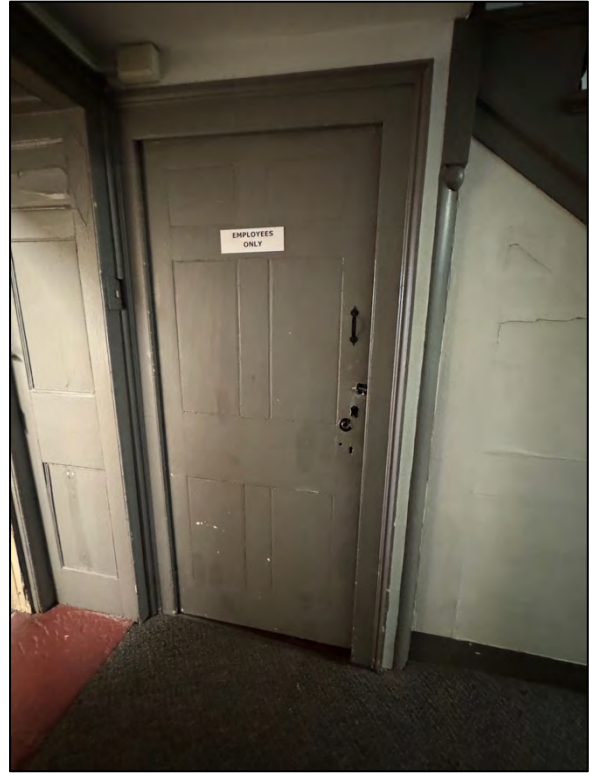
Plate 178. Door to the basement, facing north.
