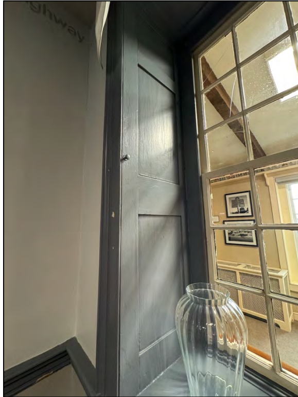
Plate 168. Detail of pocket shutters, facing west.
