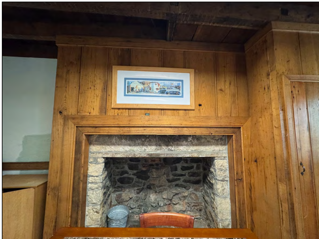
Plate 152. Detail of the hearth wall, facing north.
