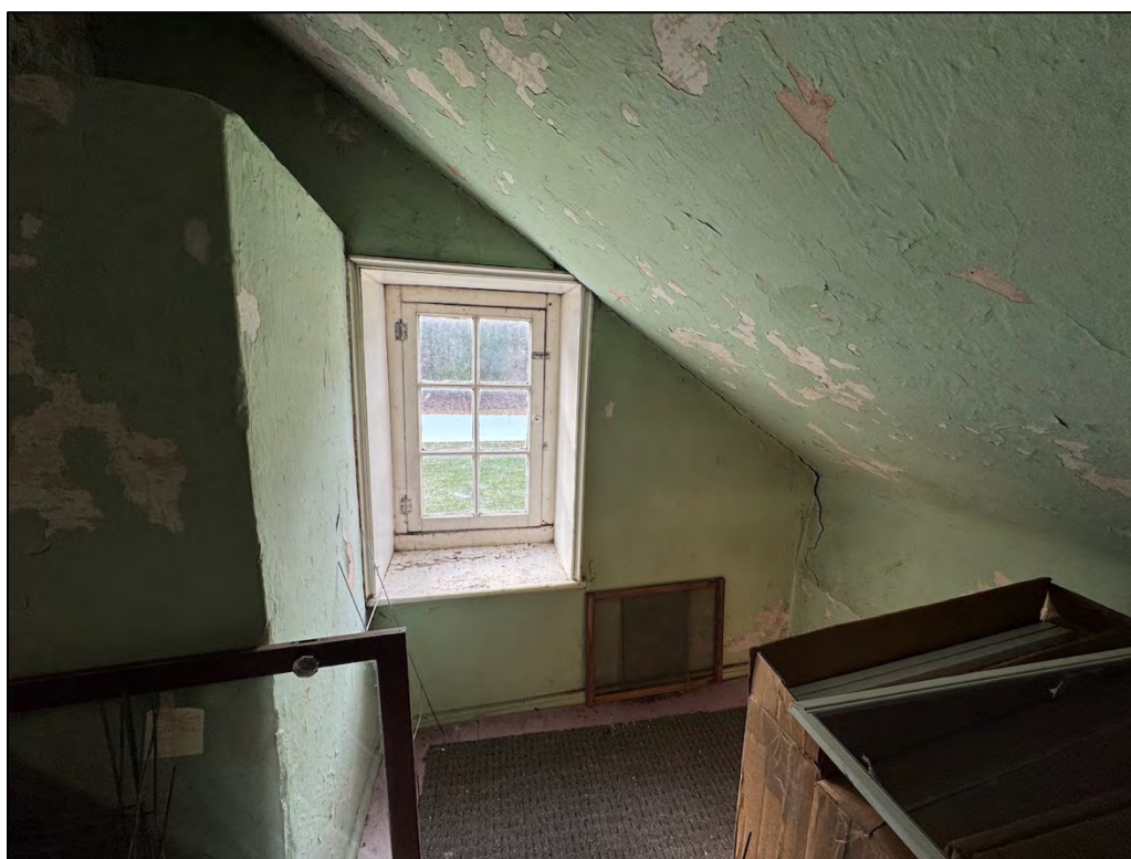
Plate 322. Room 18, south wing upper storage area, facing south.
