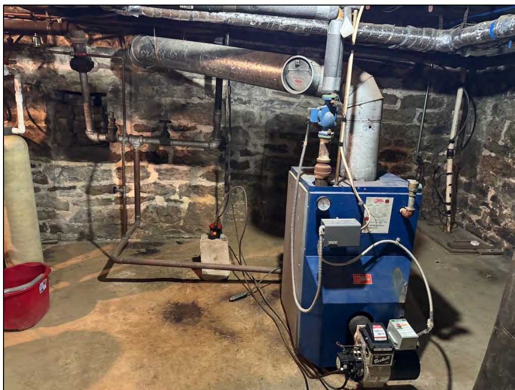
Plate 126. North wall, facing north. Note sump pump in the right corner.
