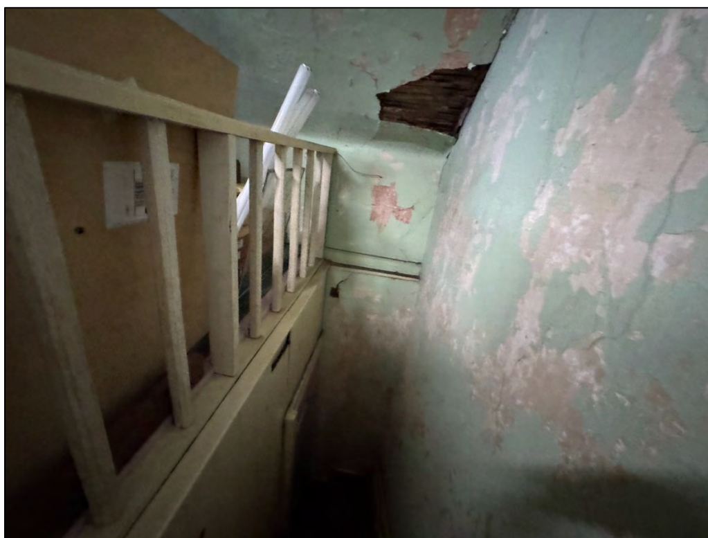
Plate 330. Room 18, south wing upper storage area, facing west (stairwell).
