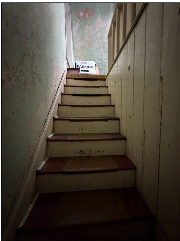
Plate 333. Stairs leading to Room 18 from Room 10 (Ship Room).
