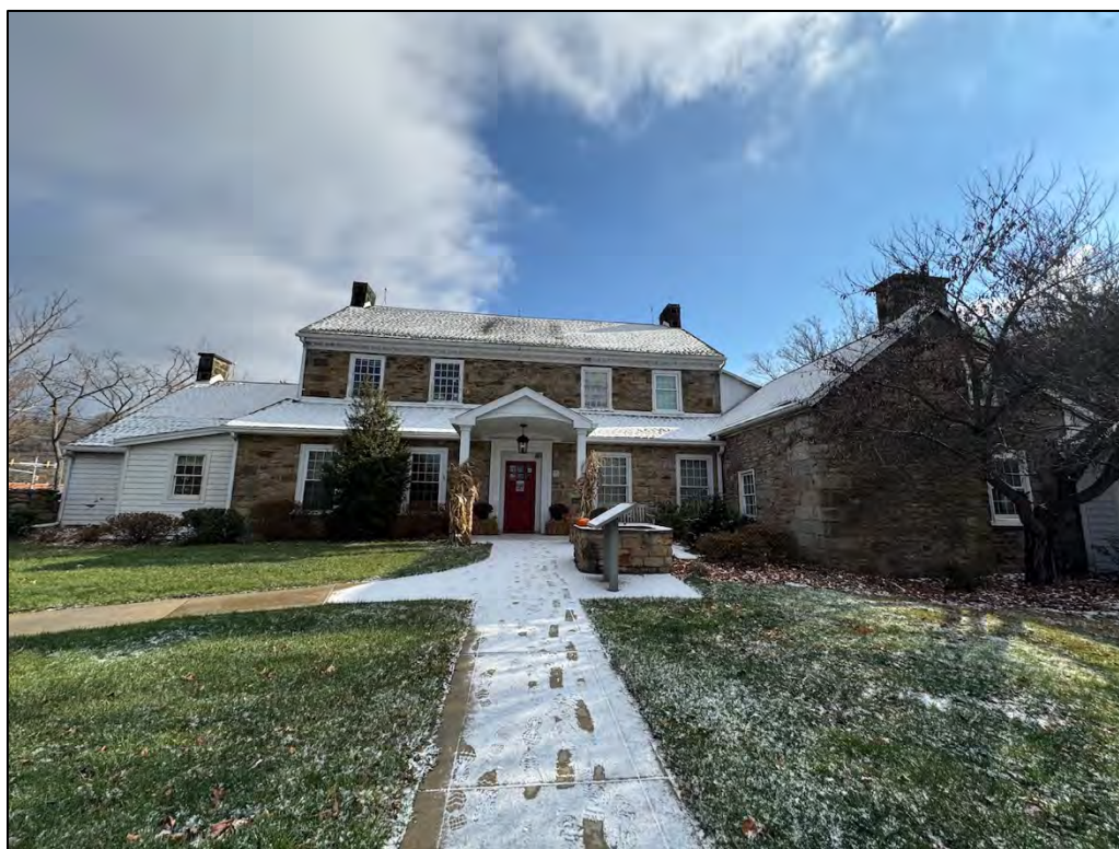
Plate 119. Typical west elevation windows. First level windows are all vinyl except for the two to the right of the door. On the second level, the fenestration generally consists of replacement wood windows with a single vinyl window to the right (W2-7).
