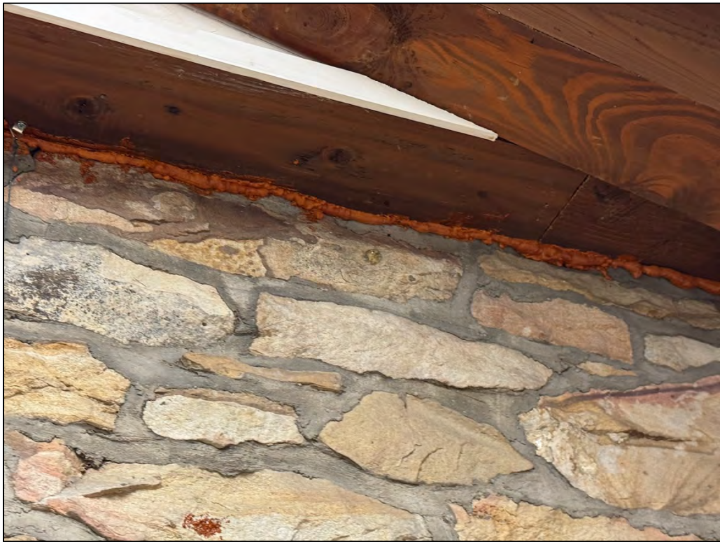
Plate 140. Connection between porch/lobby roof and the former tavern/tot room, infilled with spray foam, facing south.
