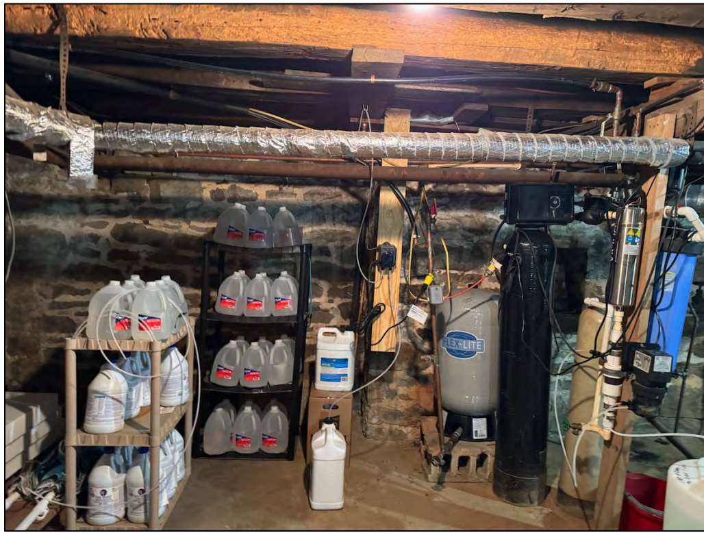
Plate 127. Basement, facing north.
