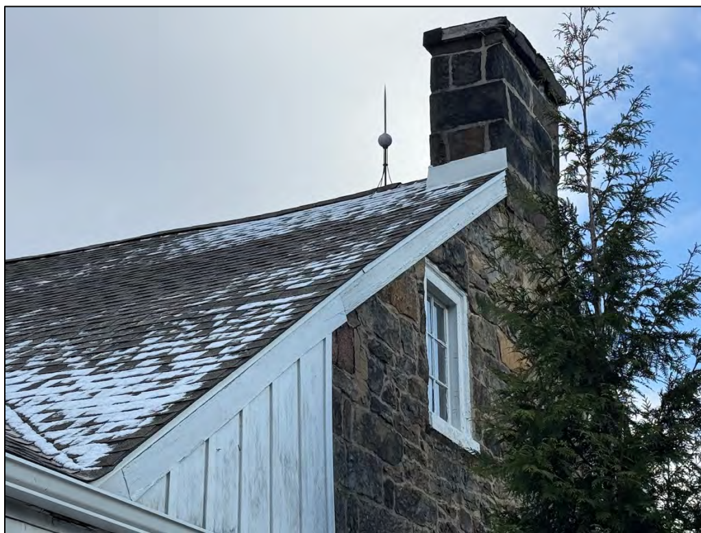
Plate 67. Chimney 4. Facing northeast.
