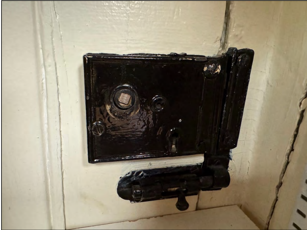
Plate 242. Detail of hardware (although of later origin). Tot Room, facing south.
