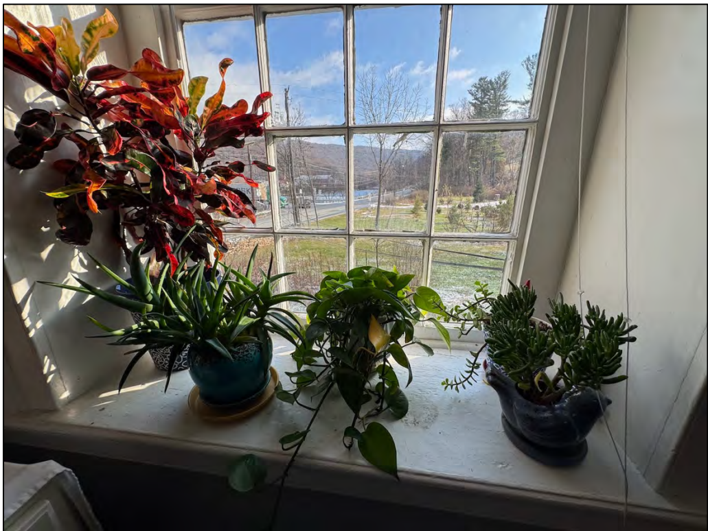
Plate 307. Wood window, facing east.
