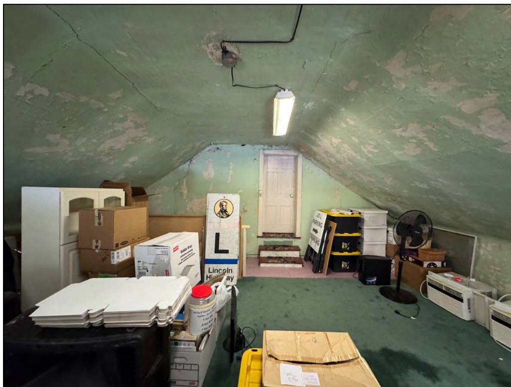
Plate 321. Room 18, south wing upper storage area, facing north.
