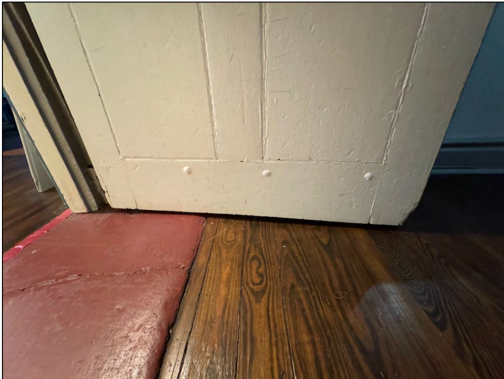
Plate 198. South elevation door, note the rivets at the bottom of the door.
