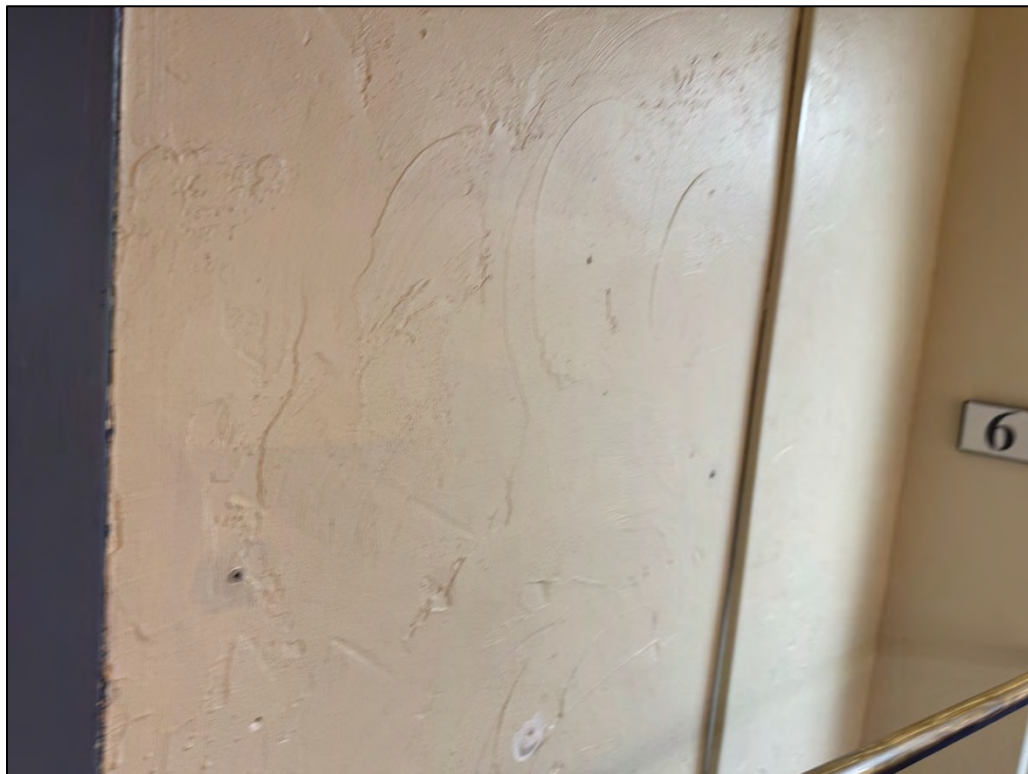
Plate 262. Typical plaster treatment in postcard hallway, facing southeast.
