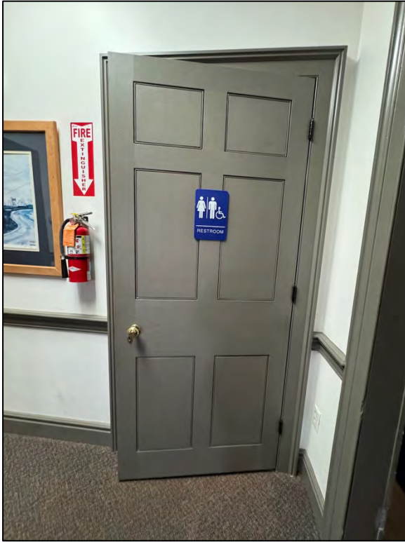
Plate 184. Modern door into First level bathroom, facing east
