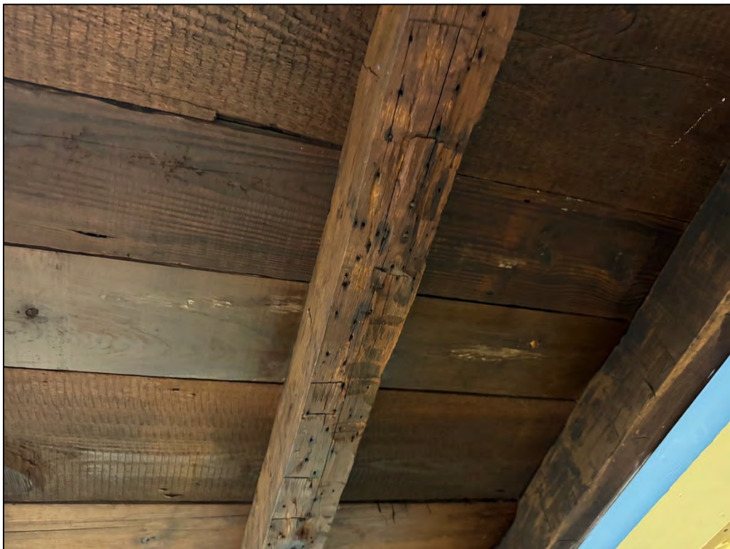
Plate 243. Detail of joists and upper-level floorboards, Tot Room.
