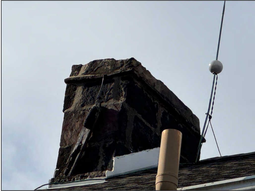
Plate 63. Chimney 3, facing west.
