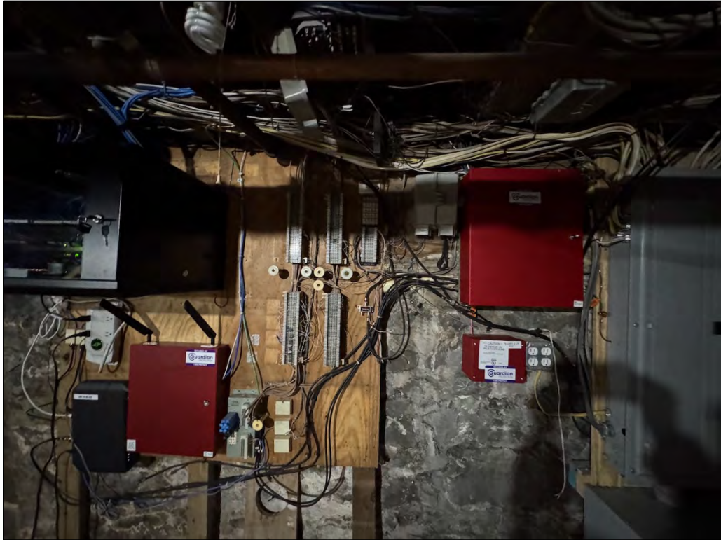
Plate 133. Electrical and telecommunication wires, on the east wall, facing east.
