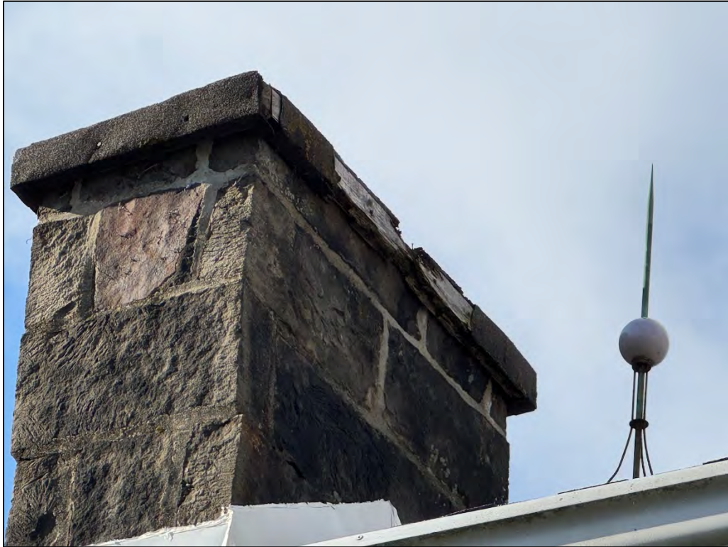
Plate 69. North and east elevation of Chimney 4, facing southwest.
