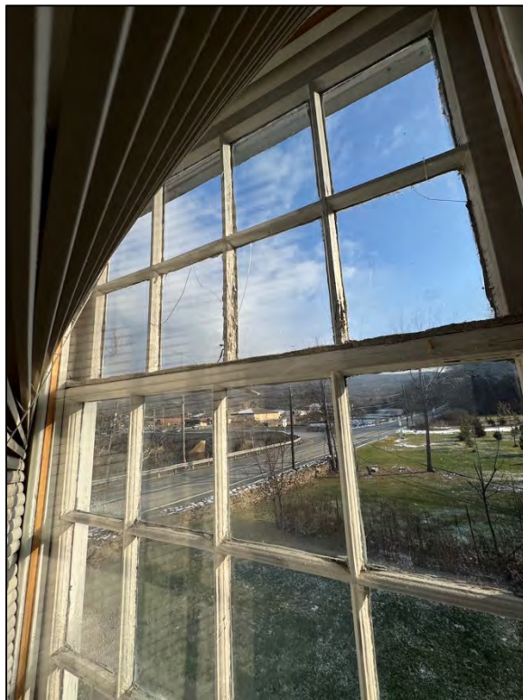
Plate 296. Upper sash of Window 2-11, facing east.
