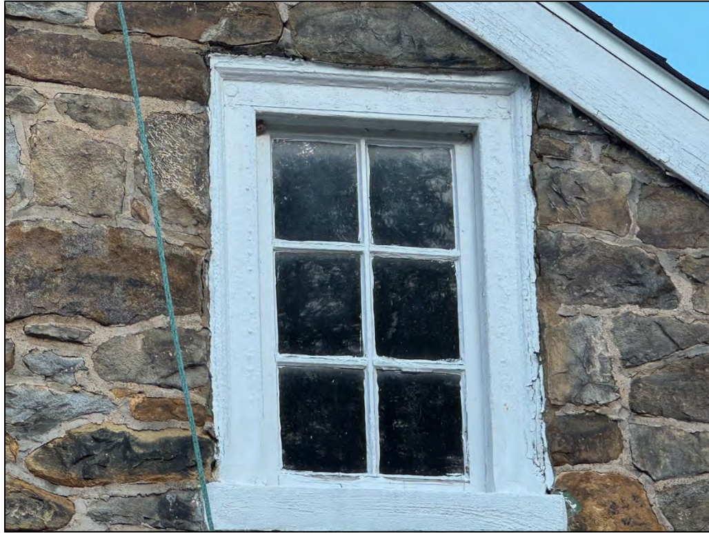
Plate 122. Typical replacement wood casement window (W2-13).
