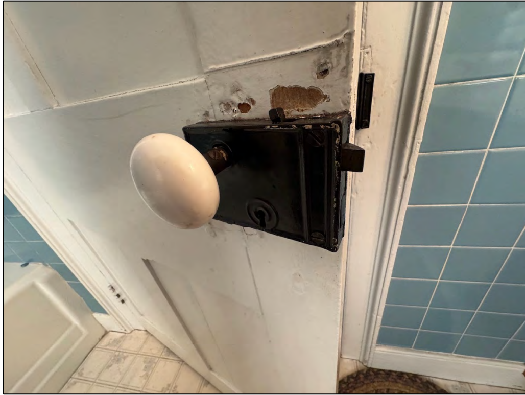
Plate 301. Detail of doorknob and hardware, facing west.
