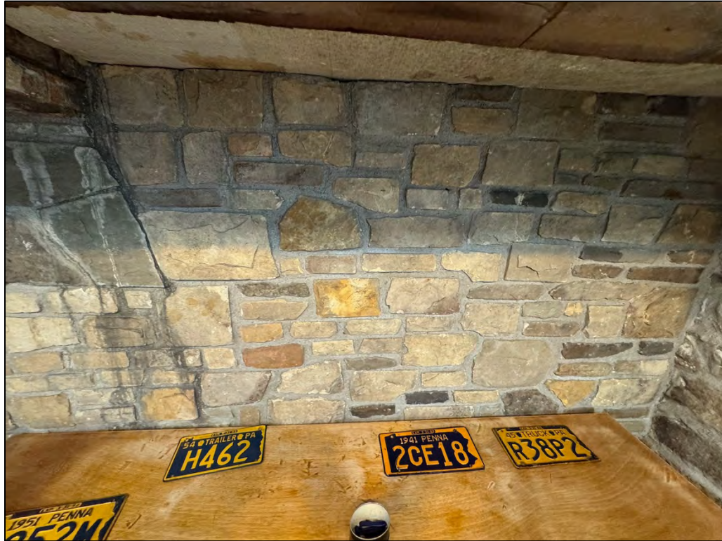
Plate 238. Replaced fireback obscures original beehive oven ghost marks, facing west. Note the insulation covering the chimney.
