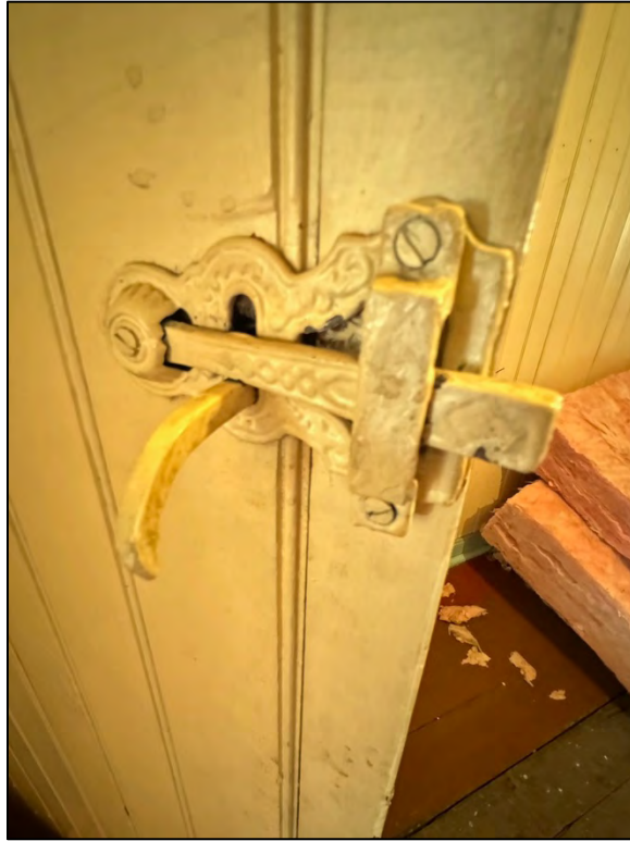
Plate 352. Hardware on door, facing west.
