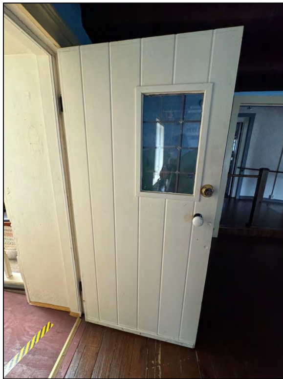
Plate 233. Entry door from Lobby/Former Porch. Facing east.
