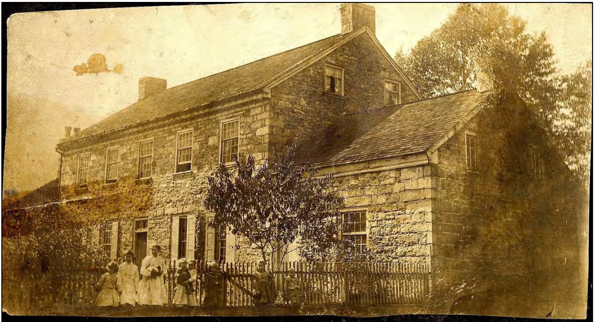
Plate 3. Johnston House, east and north elevations, ca. 1905. Courtesy the Lincoln Highway Heritage Corridor.
