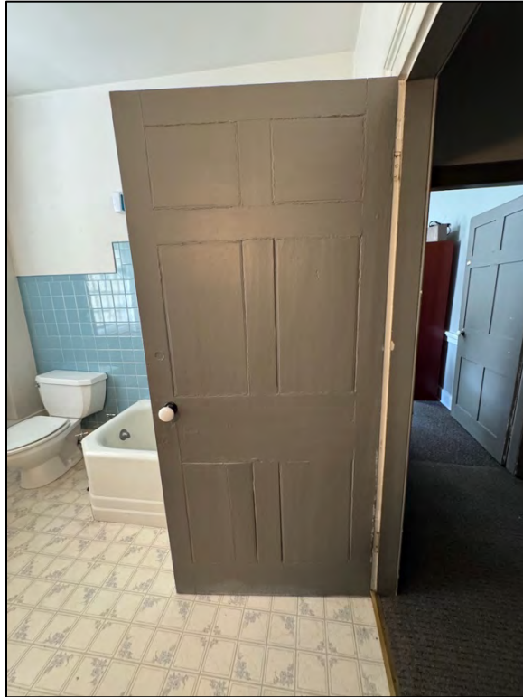
Plate 299. Detail of door, facing south.
