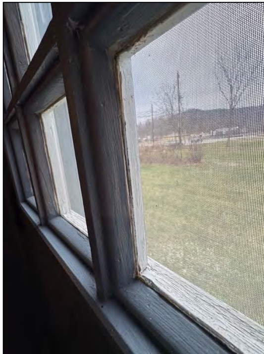
Plate 111. Detail of window, Ship Room, facing northeast.
