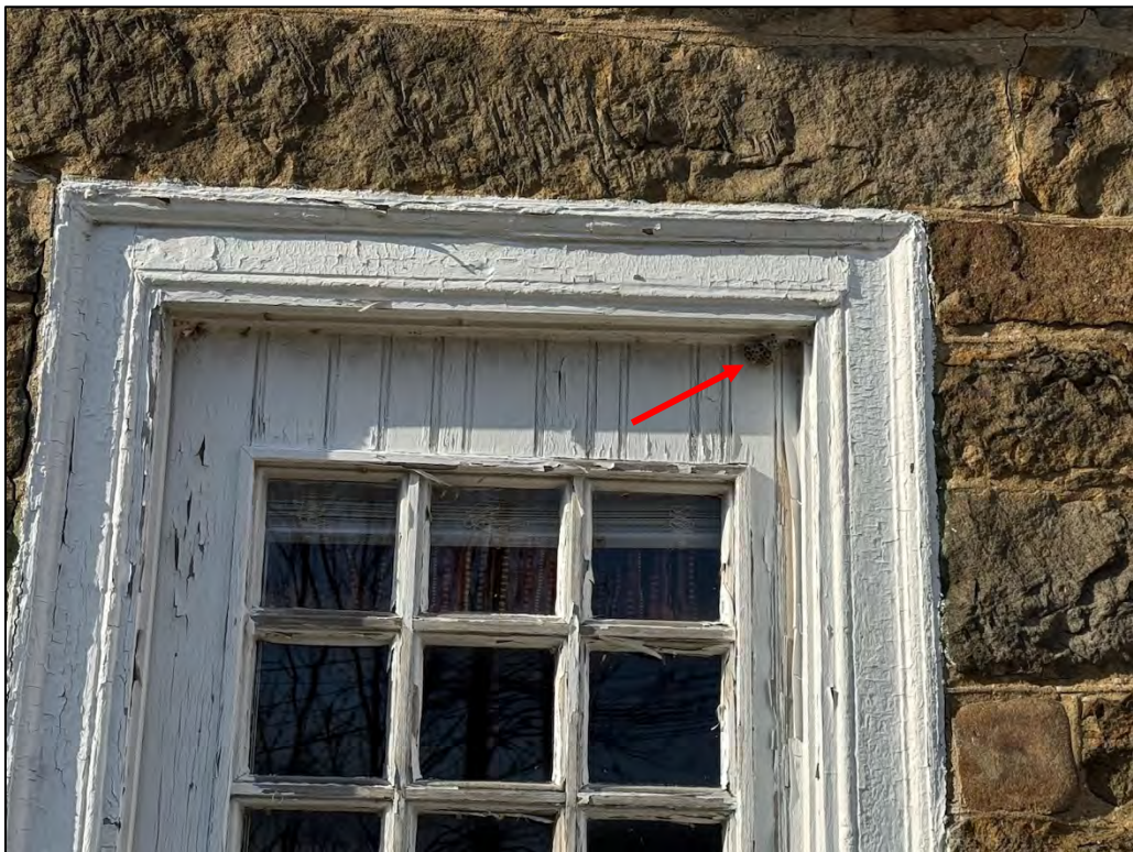
Plate 88. Northernmost door on west elevation. Note the insect nest in the upper corner.
