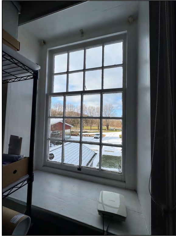
Plate 285. Typical wood window, facing west.
