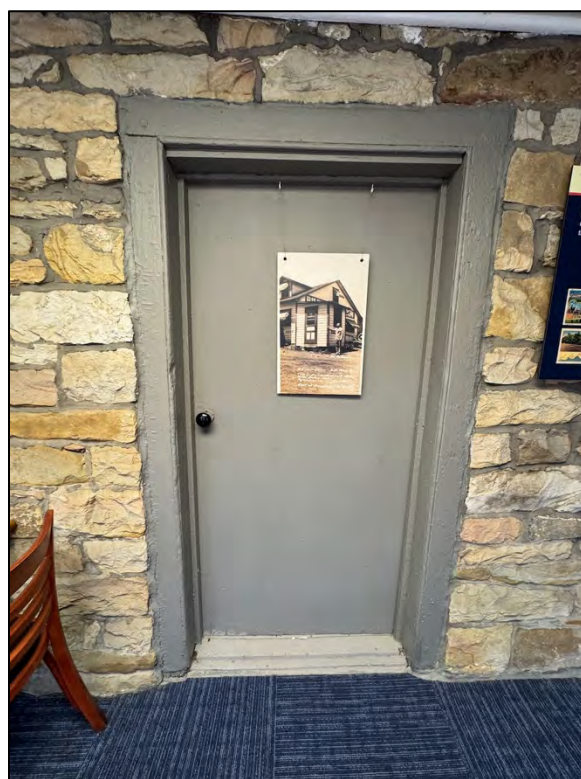
Plate 260. Opposite side of door to Tot Room, facing north.
