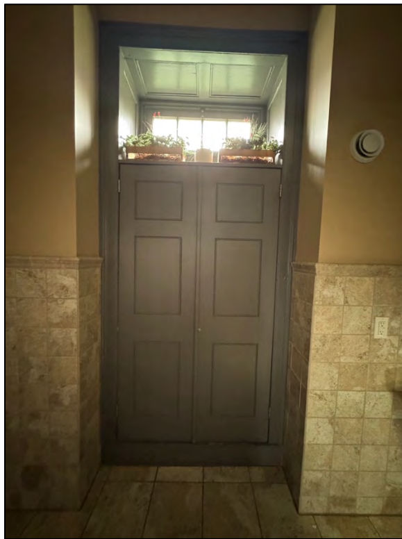
Plate 100. Interior of entry. Note the paneled ceiling.
