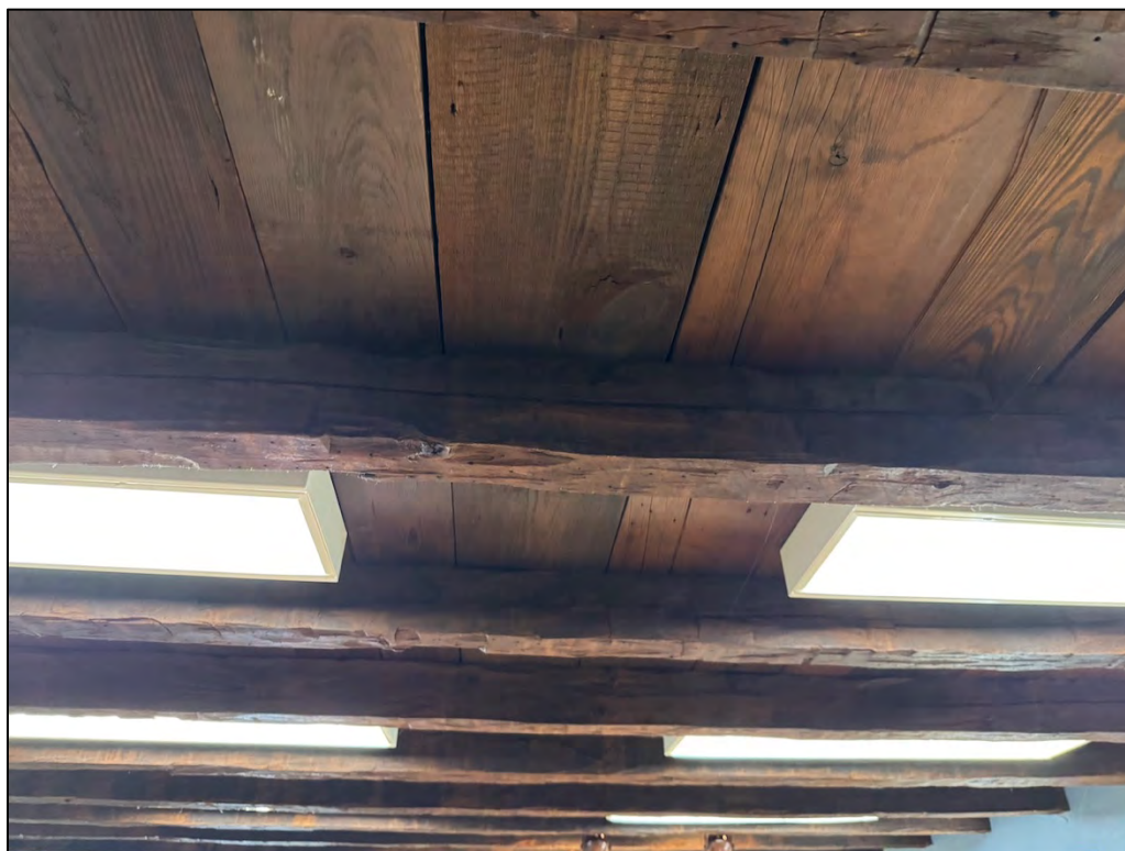
Plate 244. Typical exposed ceiling and fluorescent lights, Tot Room, facing west.
