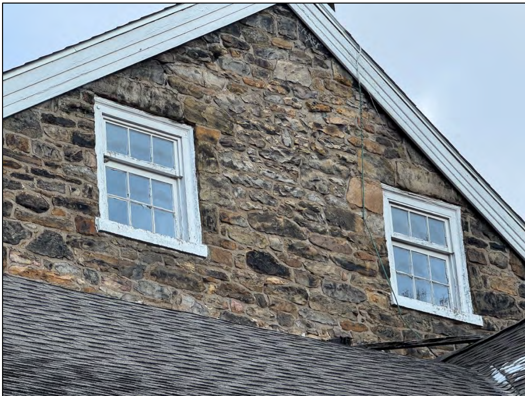
Plate 121. Typical gable end, wood windows (W3-3 and W3-4).
