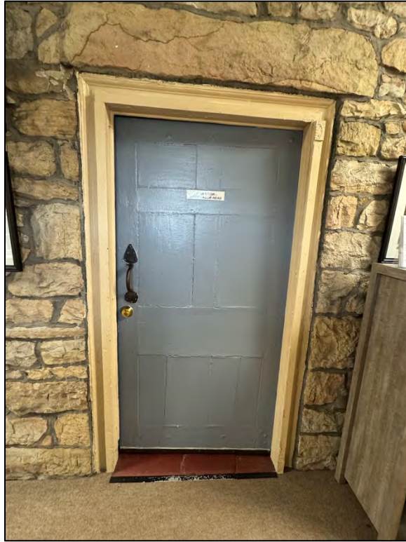
Plate 174. Doorway into the hallway from the lobby, facing east.
