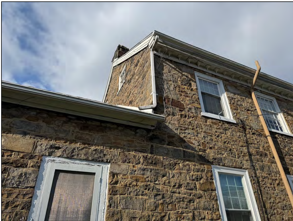
Plate 52. Typical gutter and downspout on east elevation.
