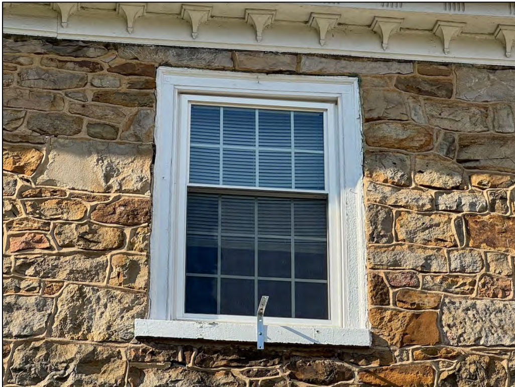
Plate 117. Typical example of vinyl replacement window, east side (W2-6).
