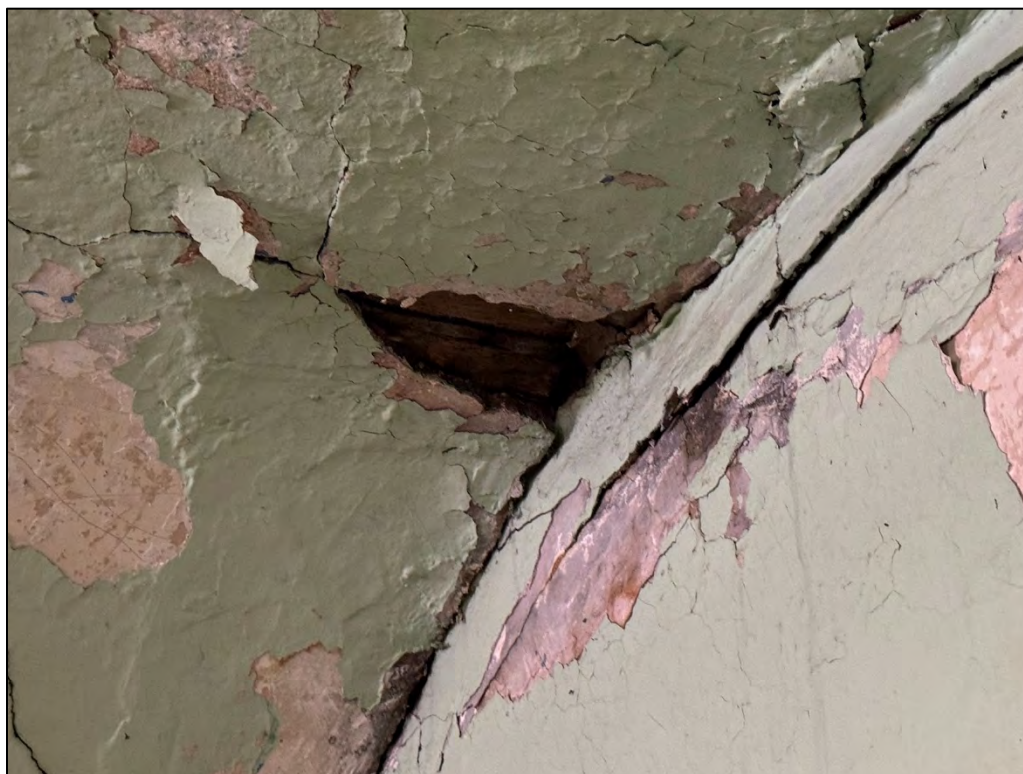
Plate 329. Room 18, south wing upper storage area, facing west.
