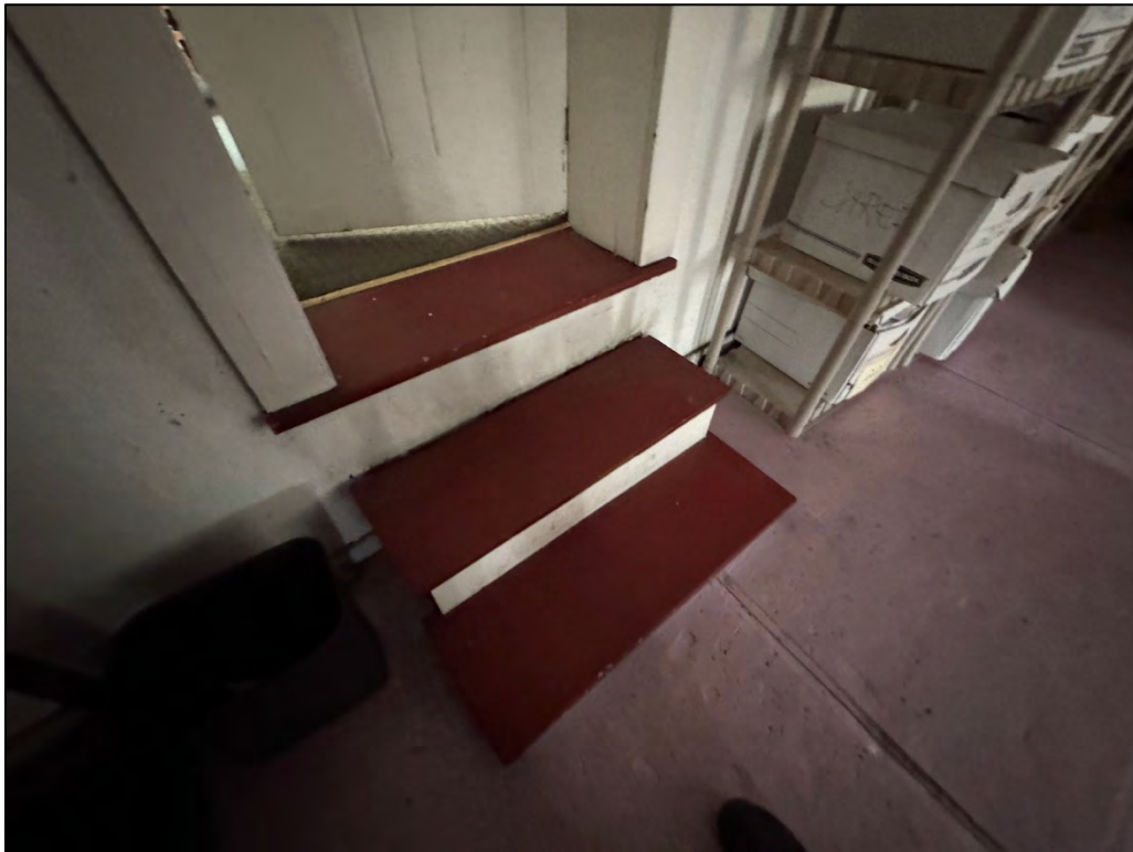
Plate 280. Entry stairs to Room 14, facing south.
