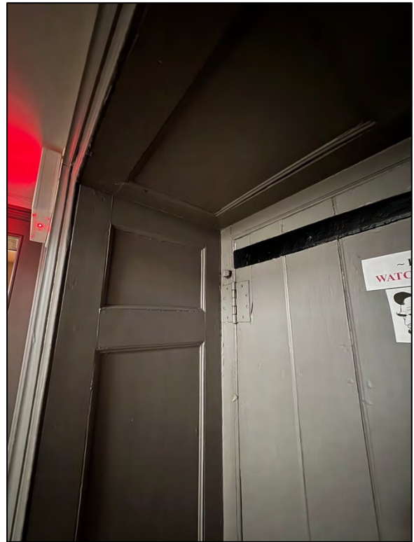
Plate 176. Interior of door frame, facing southwest.
