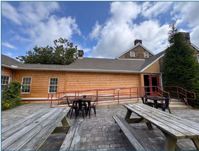
Photo 5. South elevation, facing north. Note the new siding and the HVAC piping.
