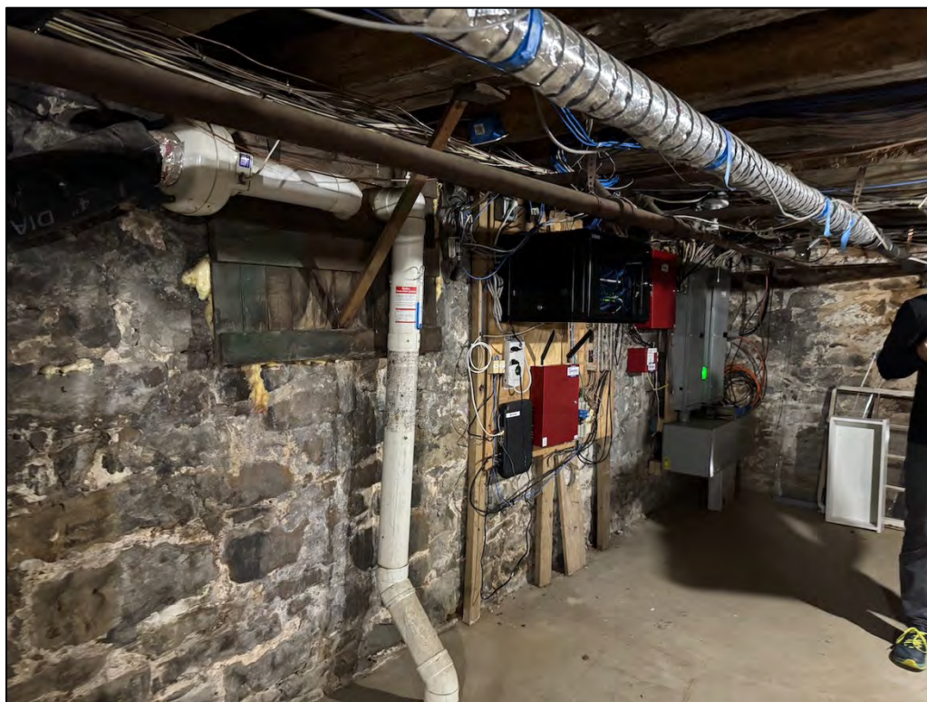
Plate 37. Foundation wall, facing southeast
