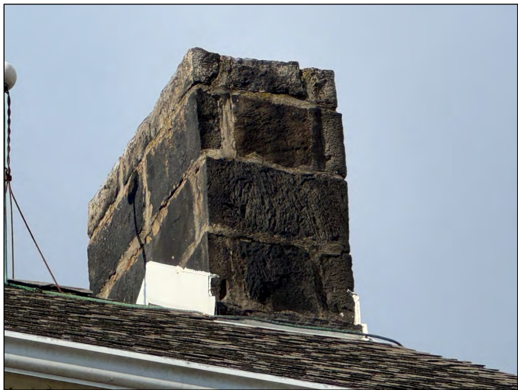
Plate 60. Chimney 2, facing northwest.
