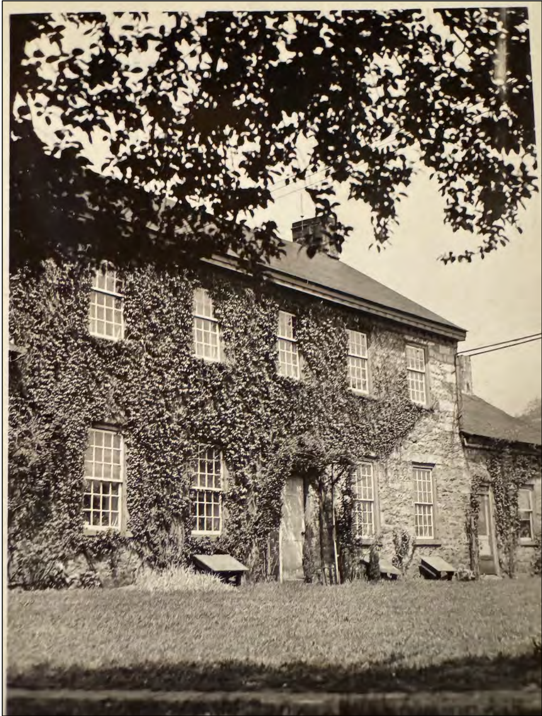
Plate 10. East elevation, ca. 1930. Photo by Charles Stoltz. Courtesy of Heinz History Center.
