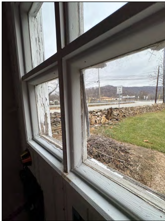
Plate 92. Interior of window, showing the thickness of the muntins, facing northeast.
