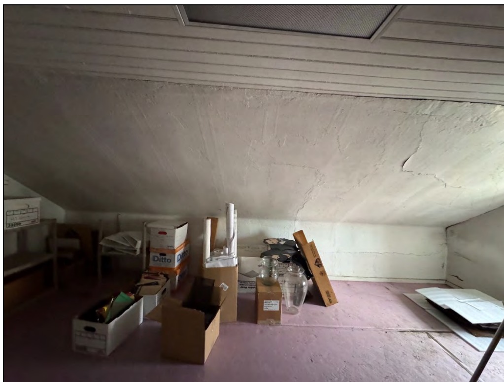
Plate 267. Upper level, northern wing, facing west.
