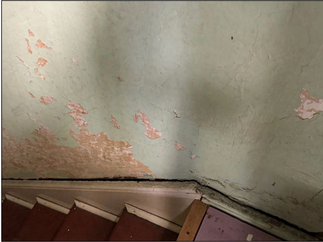
Plate 327. Room 18, south wing upper storage area, facing northwest.
