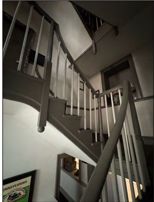
Plate 187. Stairway balustrade with dropped pendants, and turned stair knobs, facing southwest.
