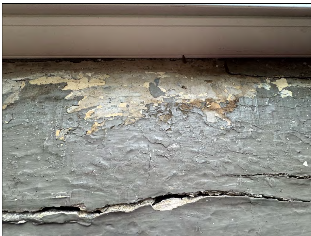
Plate 209. Window 1-16, facing east.
