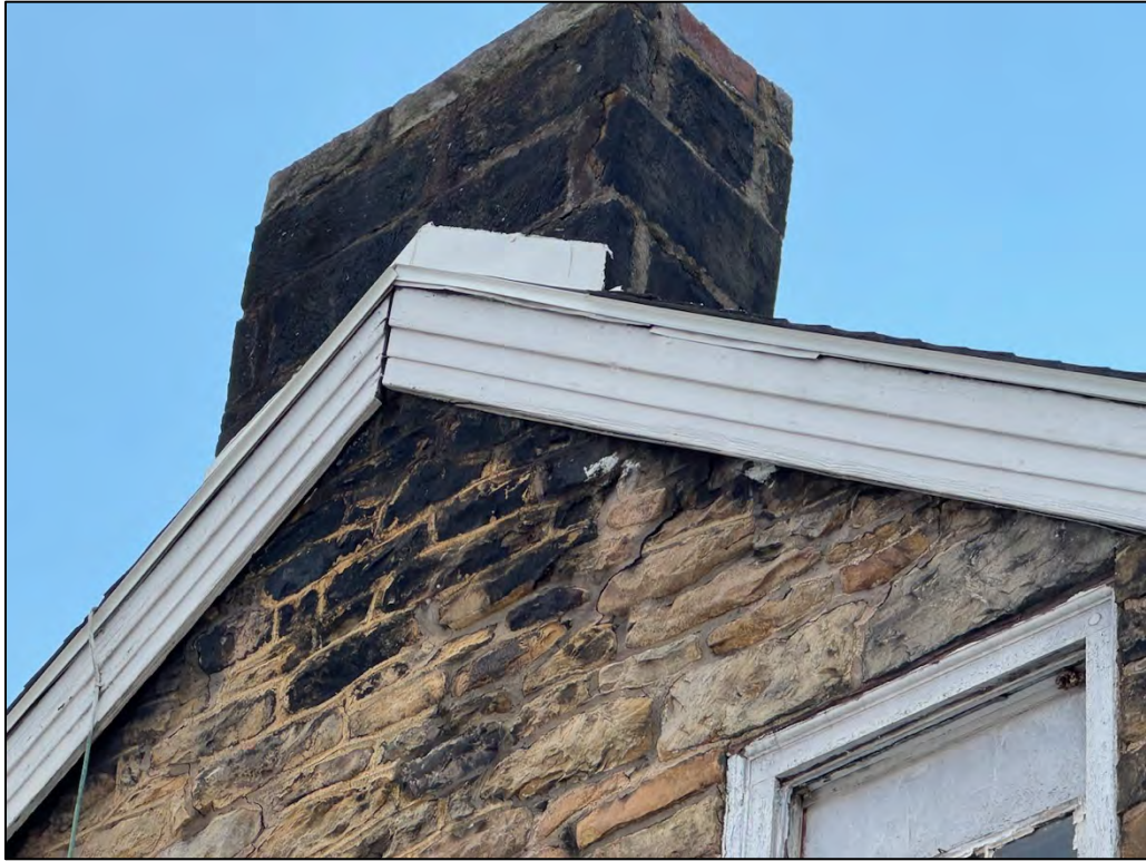
Plate 61. Chimney 2, facing southeast.
