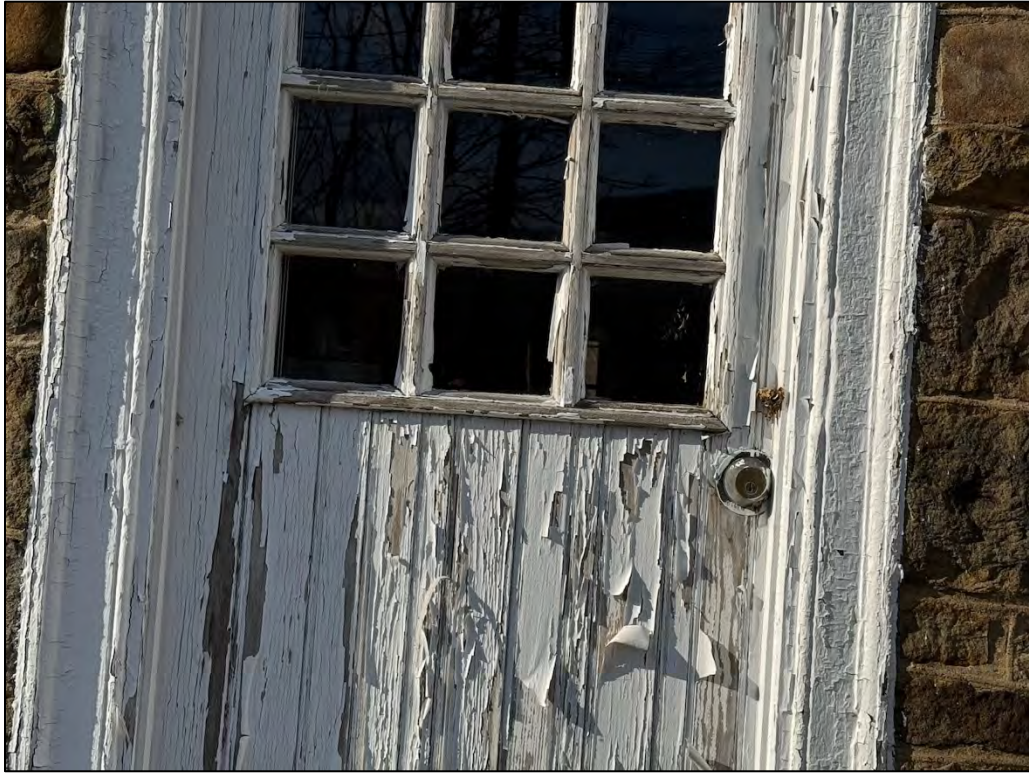
Plate 87. Northernmost door on west elevation. The door handle has been replaced with a keyed lock.
