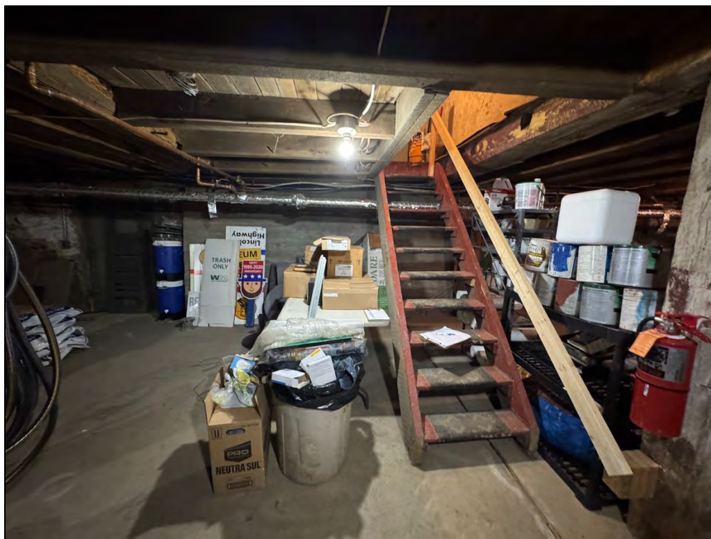
Plate 125. Room 1, facing west. The different type of support joist suggests this staircase was added later (mid-late 19 th c.).
