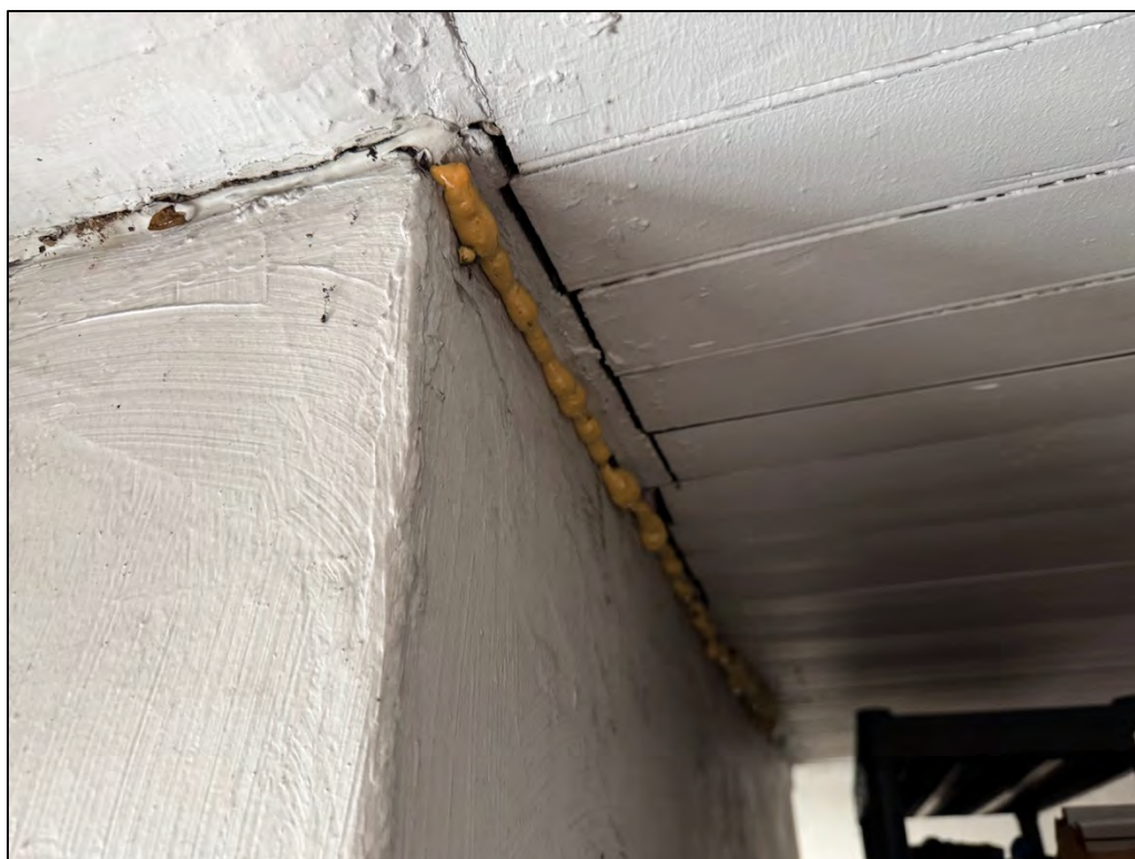
Plate 278. Room 13, detail of spray foam at the chimney/ceiling junction.
