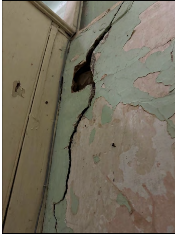
Plate 331. Room 18, south wing upper storage area, facing west (stairwell).
