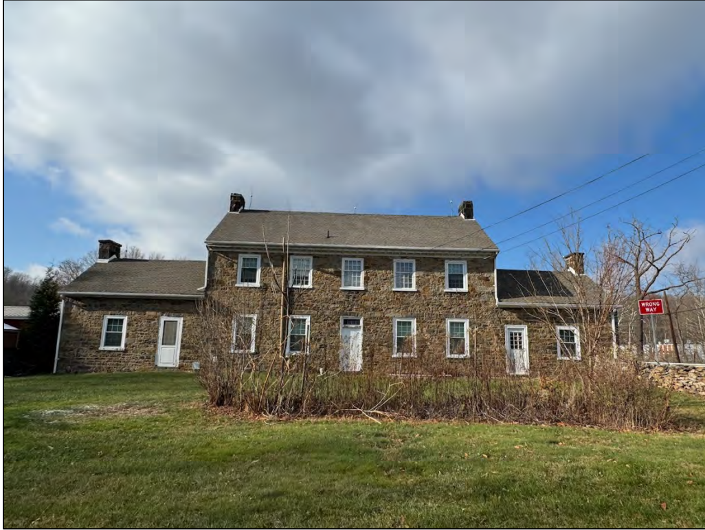
Plate 116. Representative windows, east elevation. All first-floor windows are vinyl. The three central, second story windows are wood replacement units flanked by vinyl windows.
