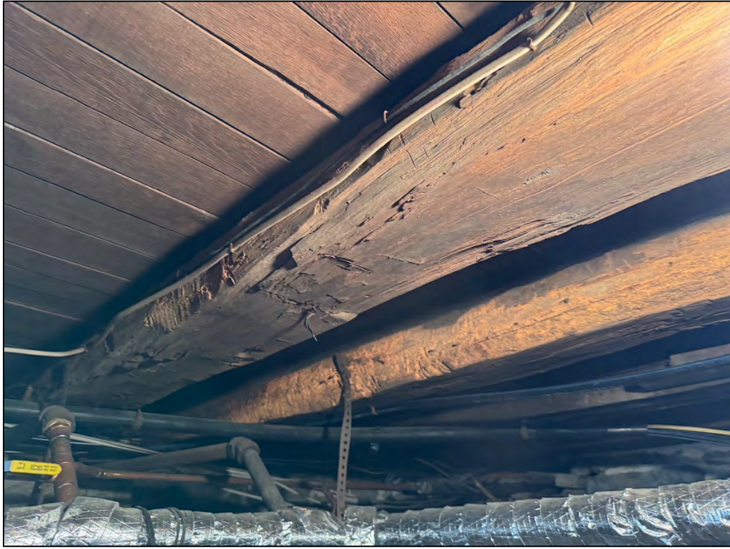
Plate 129. Original beams, facing north.
