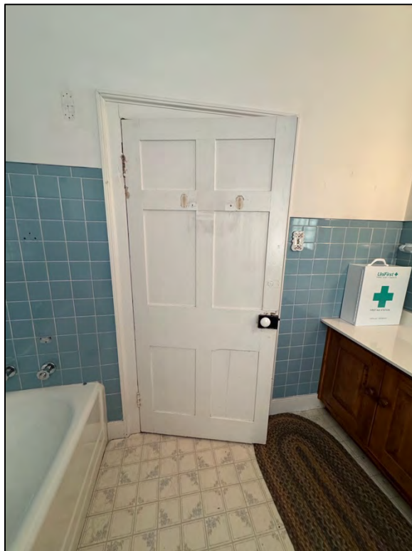
Plate 300. Detail of door, facing west.
