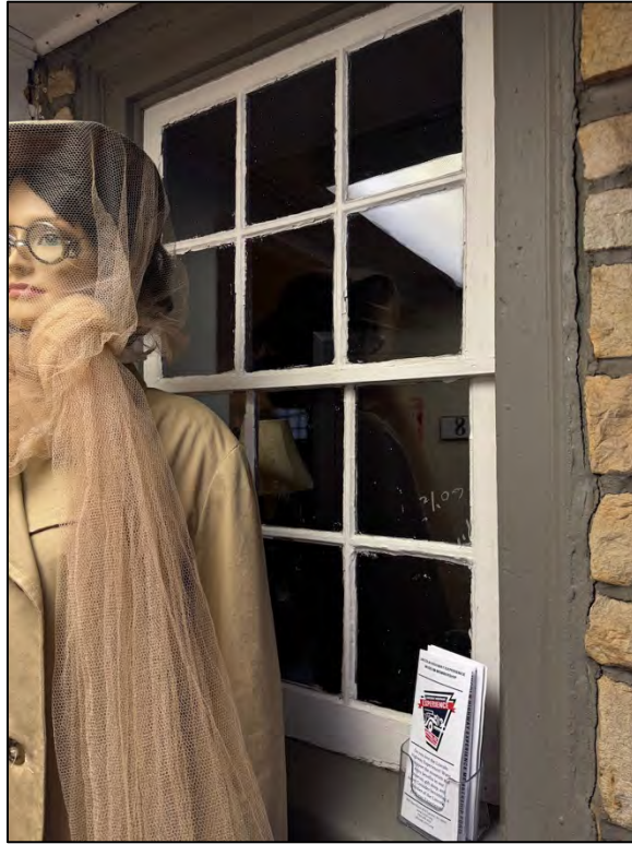
Plate 227. Typical wood window, view from hallway to Ship Room.
