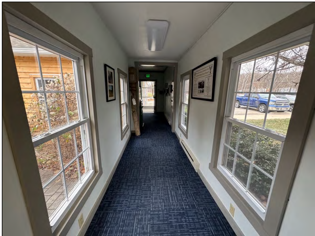
Plate 256. Hallway to Gantz Gallery, facing west.
