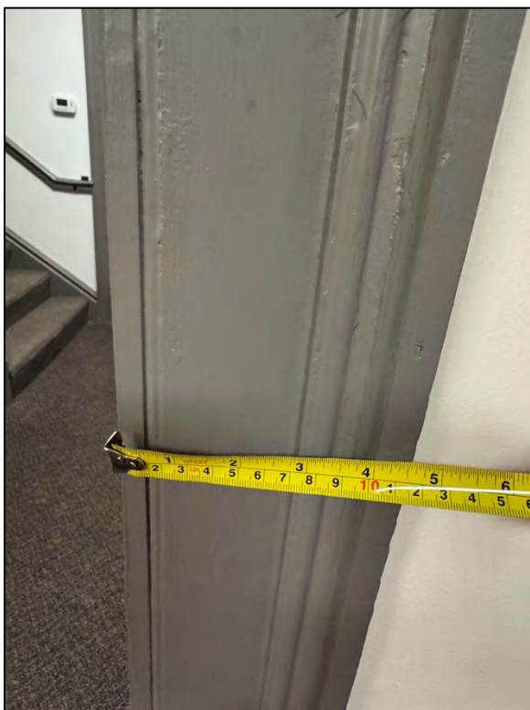
Plate 214. Door casing, facing north.
