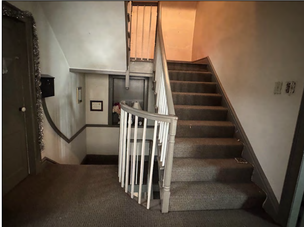
Plate 189. Stairwell, second level, facing west.
