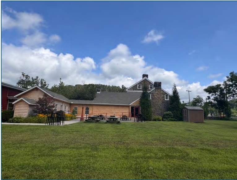
Photo 4. South elevation, facing north. Note the new siding.
