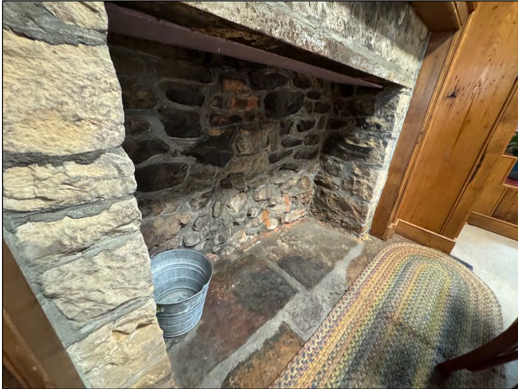
Plate 153. Room 4, facing northeast. Note the shallow fireback and enclosed chimney.
